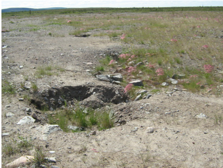
Photo 10: Minor settlement in quarry pit cover on August 5, 2009, 4 years after being filled in August, 2005.
