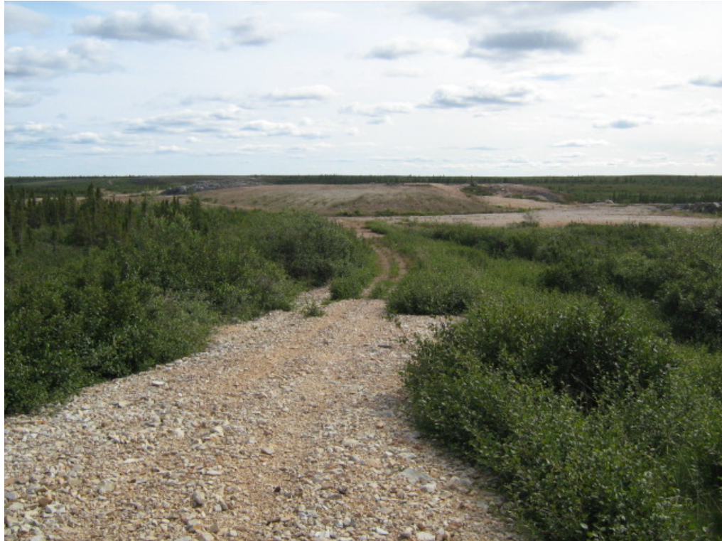
Photo 7: Encapsulated Waste Rock at Shear Lake 4 years after the application of additional seed and fertilizer. Erosion scars are visible due to being filled in with lighter coloured granular road material.
