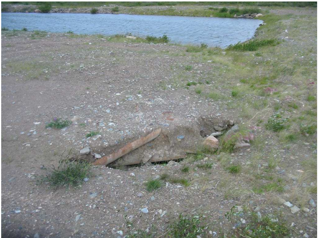
Photo 14: Subsidence at southwest corner of Quarry Pit on August 4, 2010.
