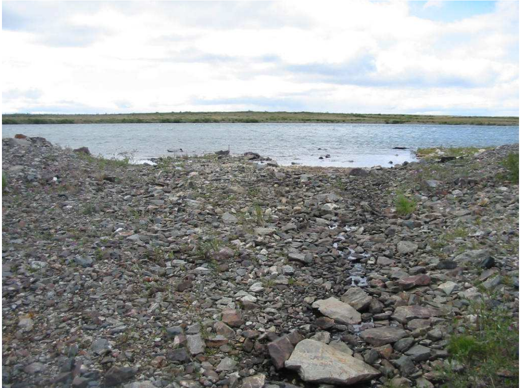
Photo 3: Tailings No.1 Pond spillway invert, looking west on August 4, 2010
