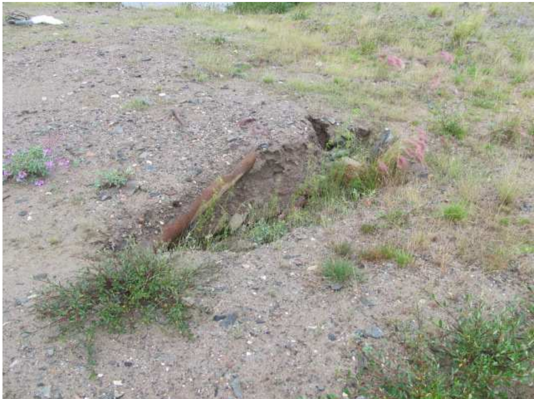
Photo 13: Subsidence at southwest corner of Quarry Pit on August 4, 2011.
