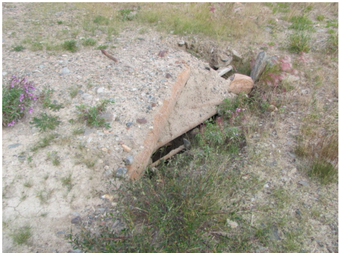
Photo 13: Subsidence at southwest corner of Quarry Pit on August 2, 2012.
