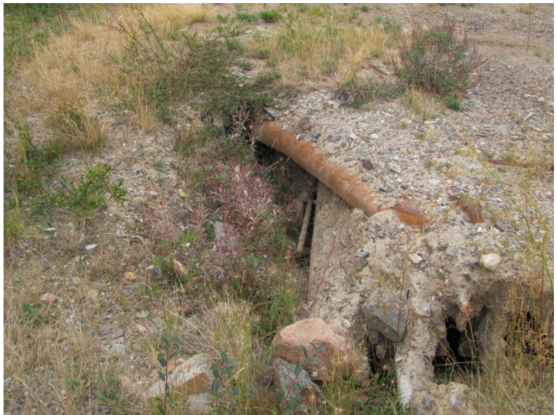
Photo 13: Subsidence at southwest corner of Quarry Pit pond on August 15, 2013.
