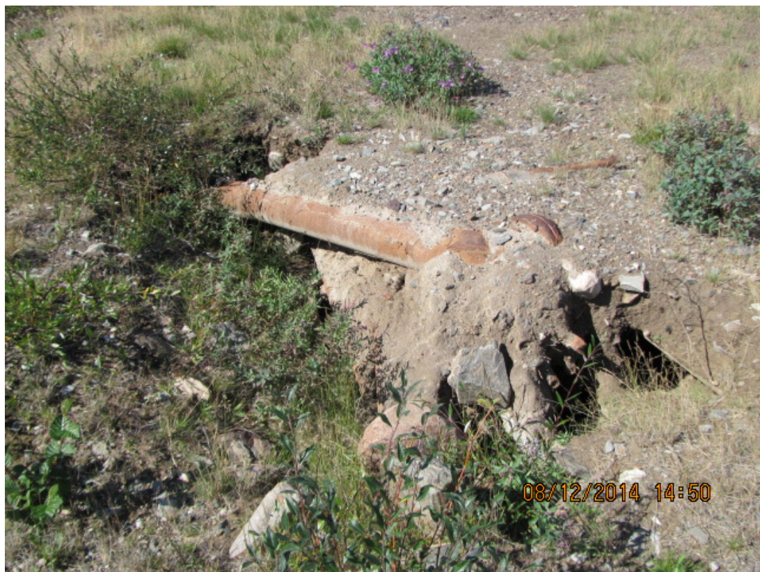
Photo 13: Subsidence at southwest corner of Quarry Pit pond on August 12, 2014.
