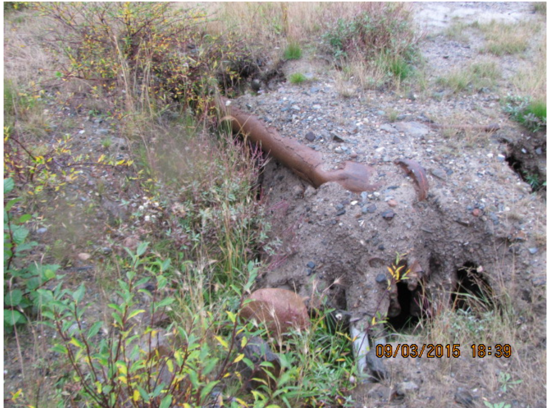
Photo 12: Subsidence area at southwest corner of of Quarry Pit pond on September 3, 2015.
