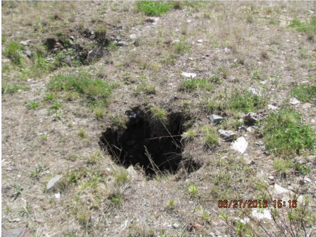
Photo 11: New subsidence area in midsection of Quarry Pit landfill cover in June 2016.
