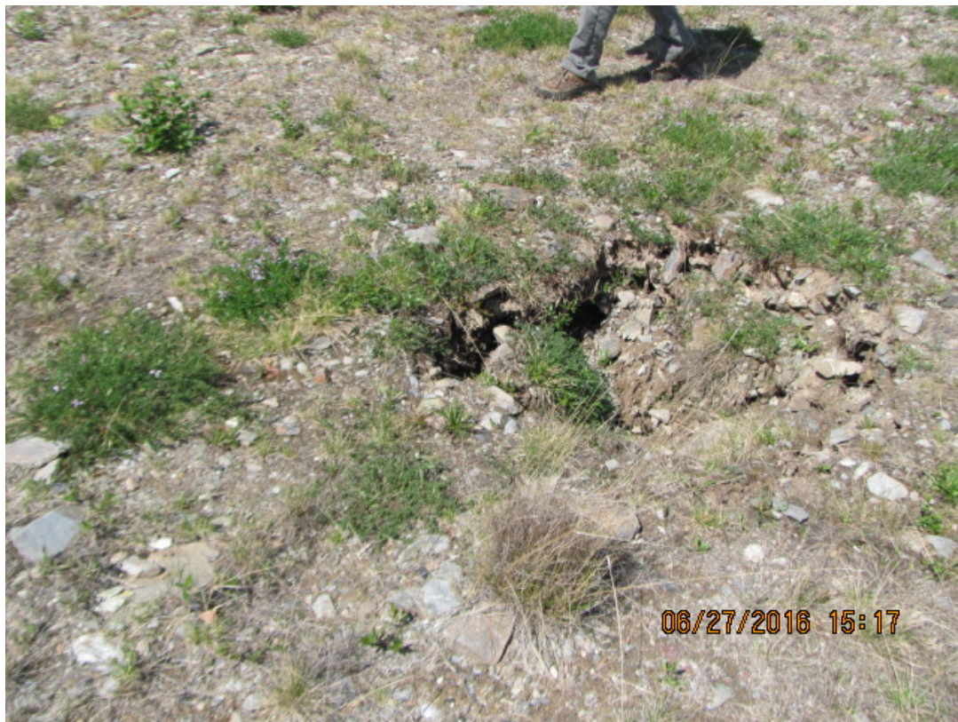
Photo 12: Subsidence at southeast corner of Quarry Pit landfill cover in June 2016.
