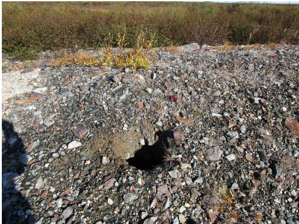
Photo 14: Small are of subsidence at B-zone Vent Raise.
