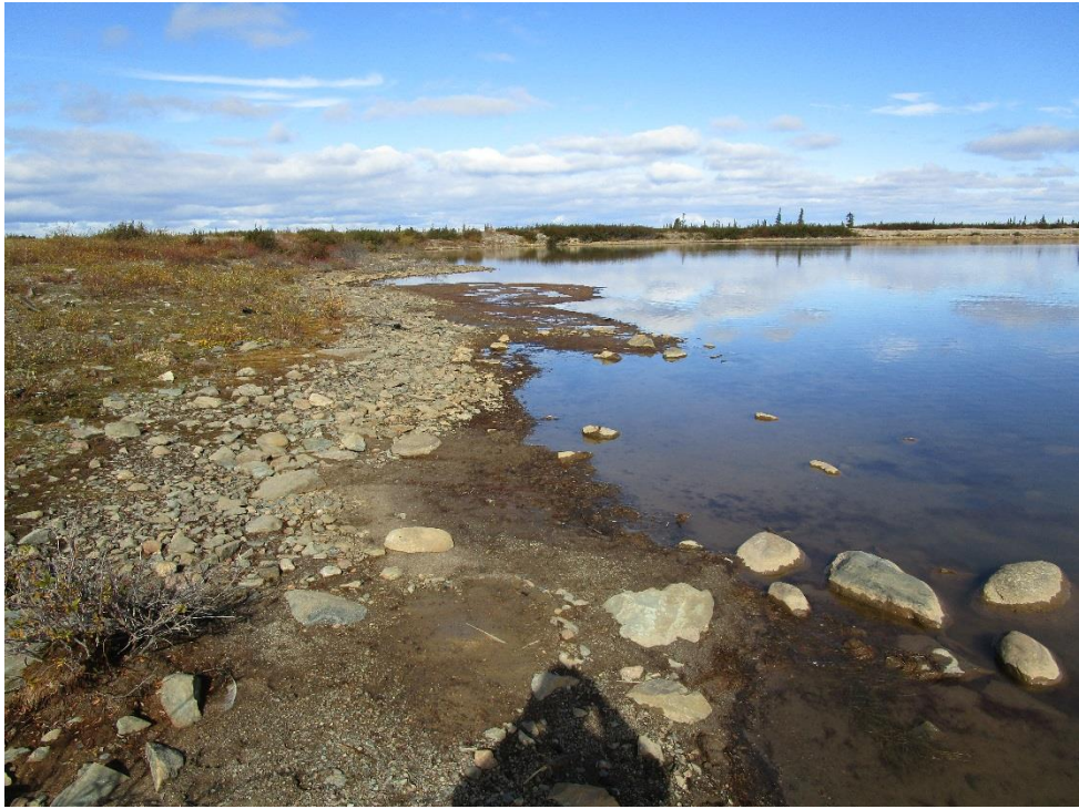
Photo 17: Exposed tailings beach on west side of pond due to low water level.
