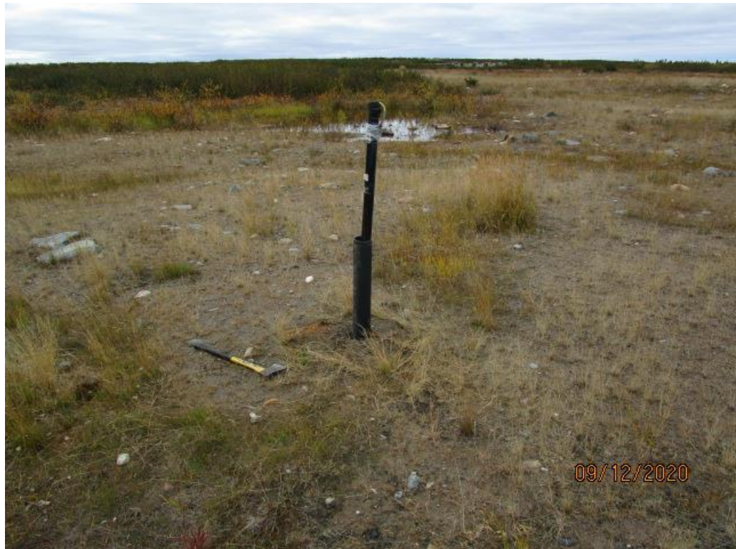
Photo 23: T1 repaired and 4-inch casing added.
