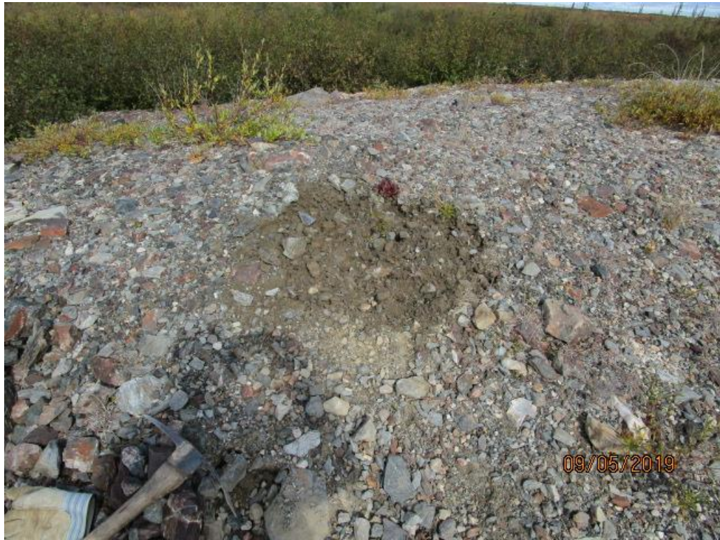
Photo 17: Small area of subsidence at B-zone Vent Raise in 2019 after filling.
