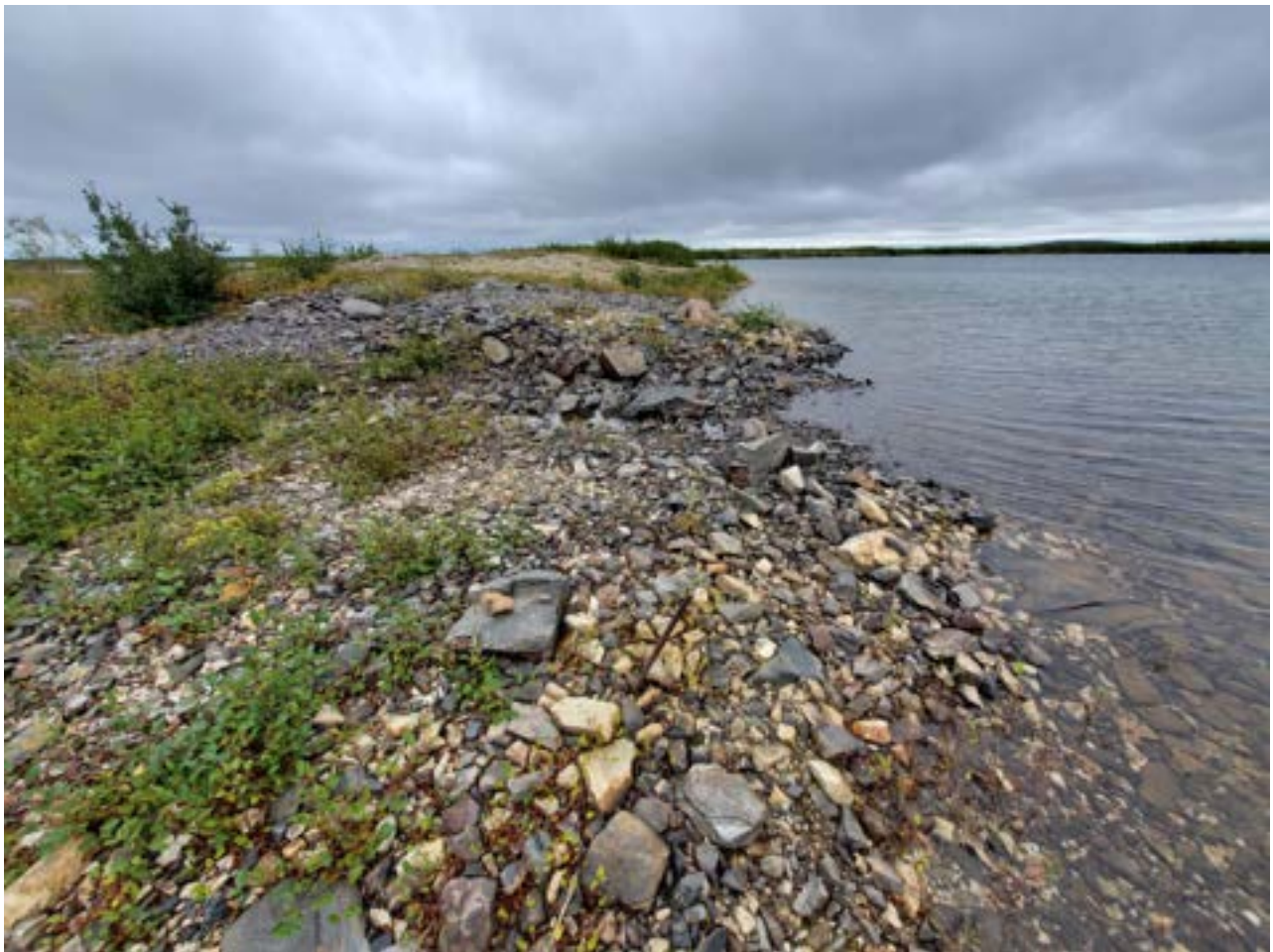
Looking across the dry outflow channel at Tailings Pond #1 (to the right)
