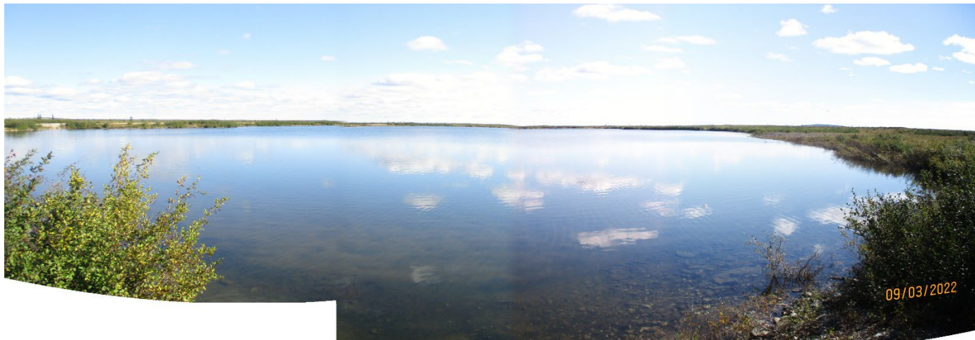
Photo 10: Tailings Pond No 1 water cover looking southeast.
