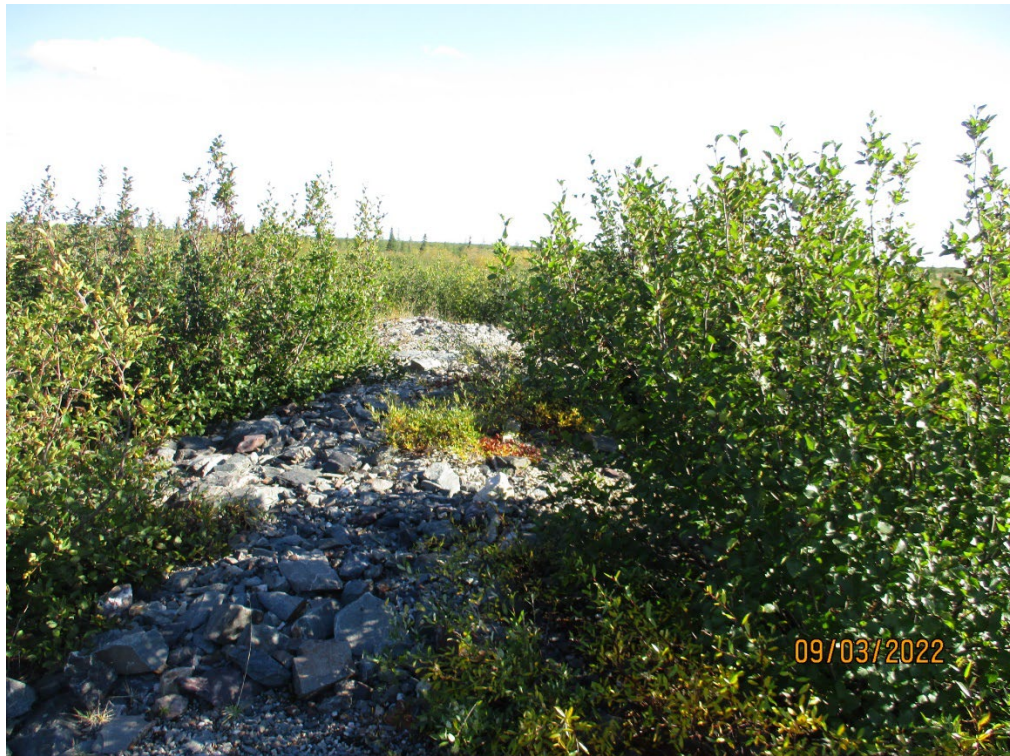
Photo 16: B-Zone raise looking west.
