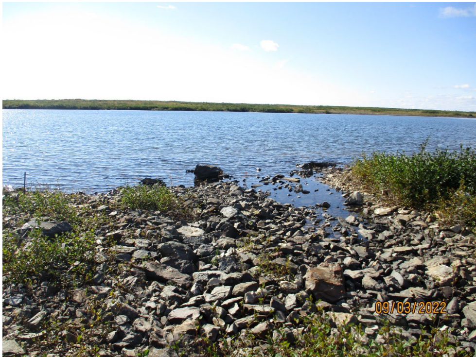
Photo 11: Tailings Pond No. 1 spillway (dry) looking upstream.
