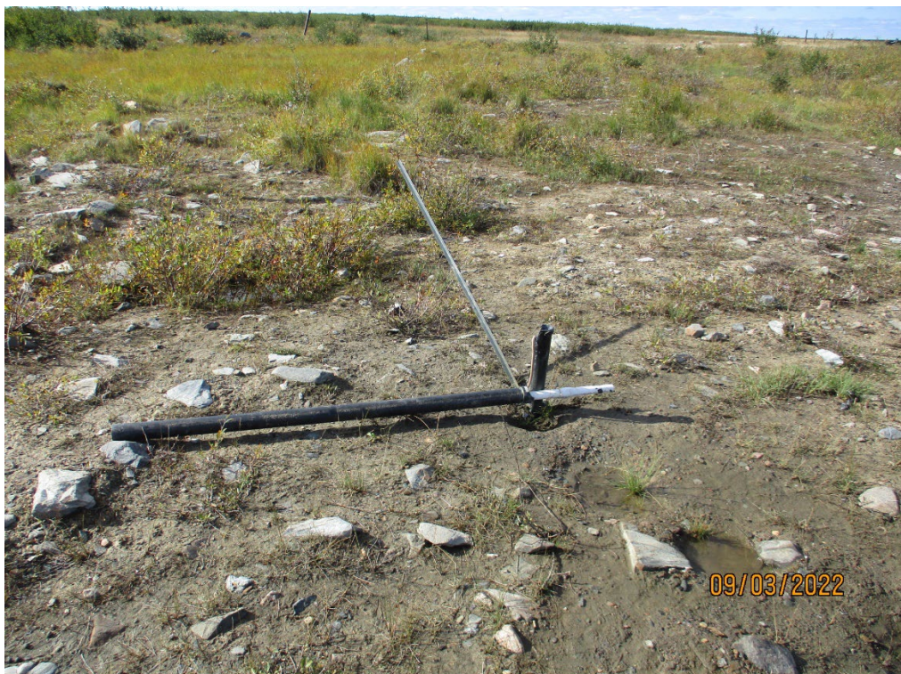
Photo 20: T3 thermistor casing damage.
