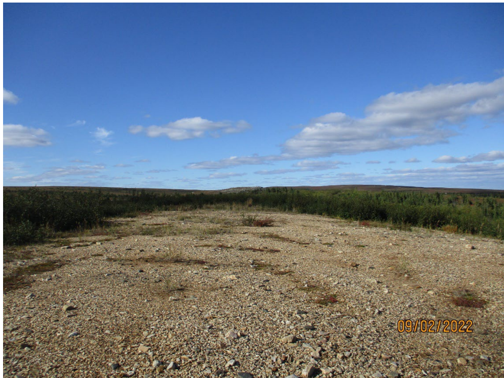
Photo 5: Encapsulated Waste Rock cover top looking north.
