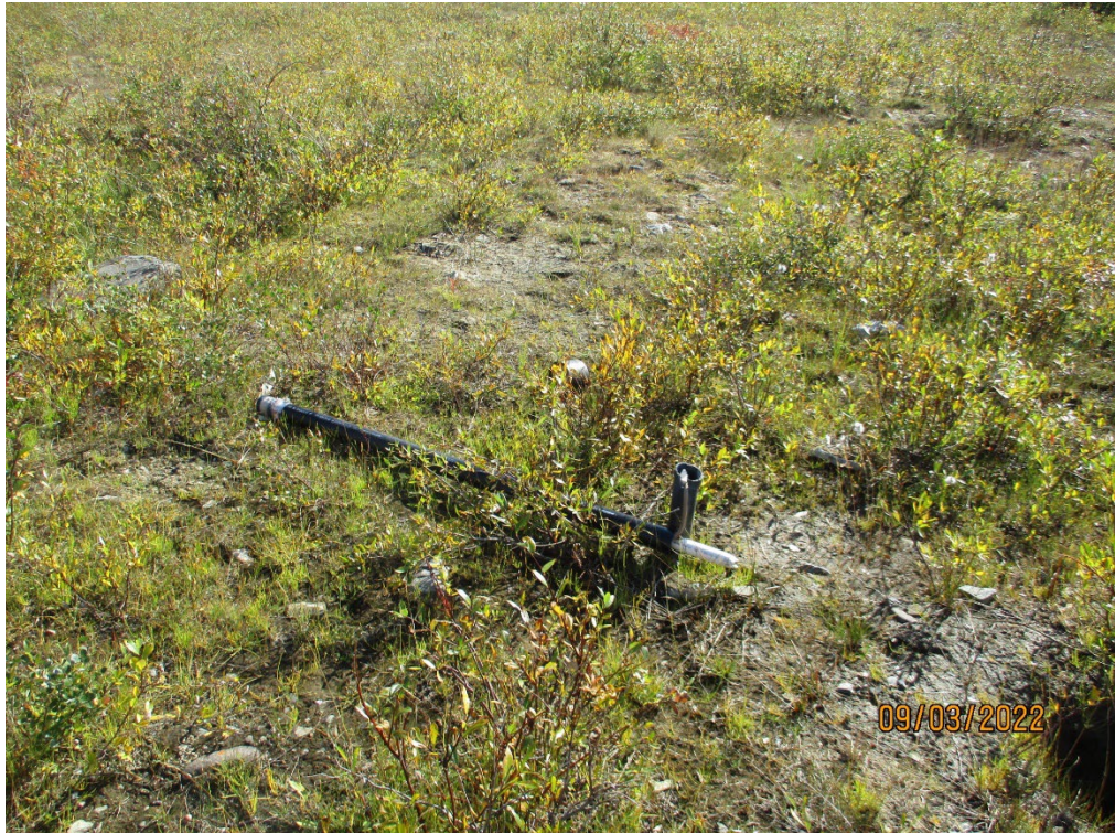
Photo 19: T2 thermistor casing damage.
