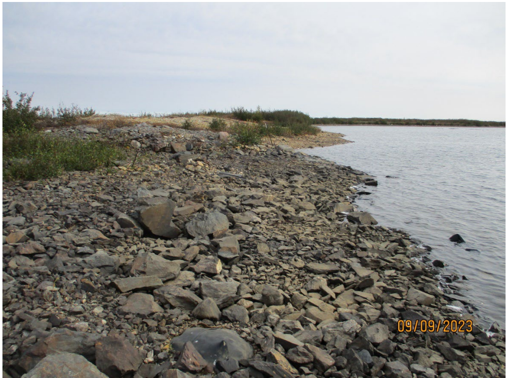
Photo 11: Tailings Pond No. 1 spillway (dry) looking south.
