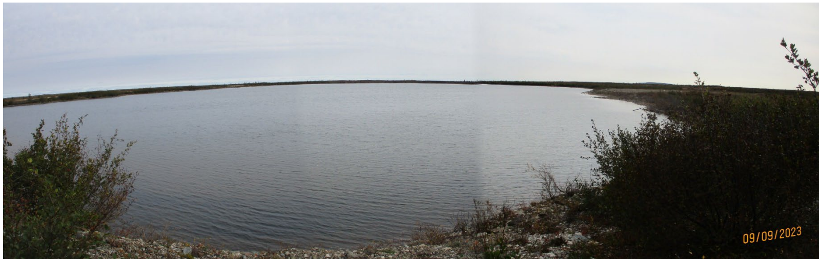
Photo 10: Tailings Pond No 1 water cover looking southeast.
