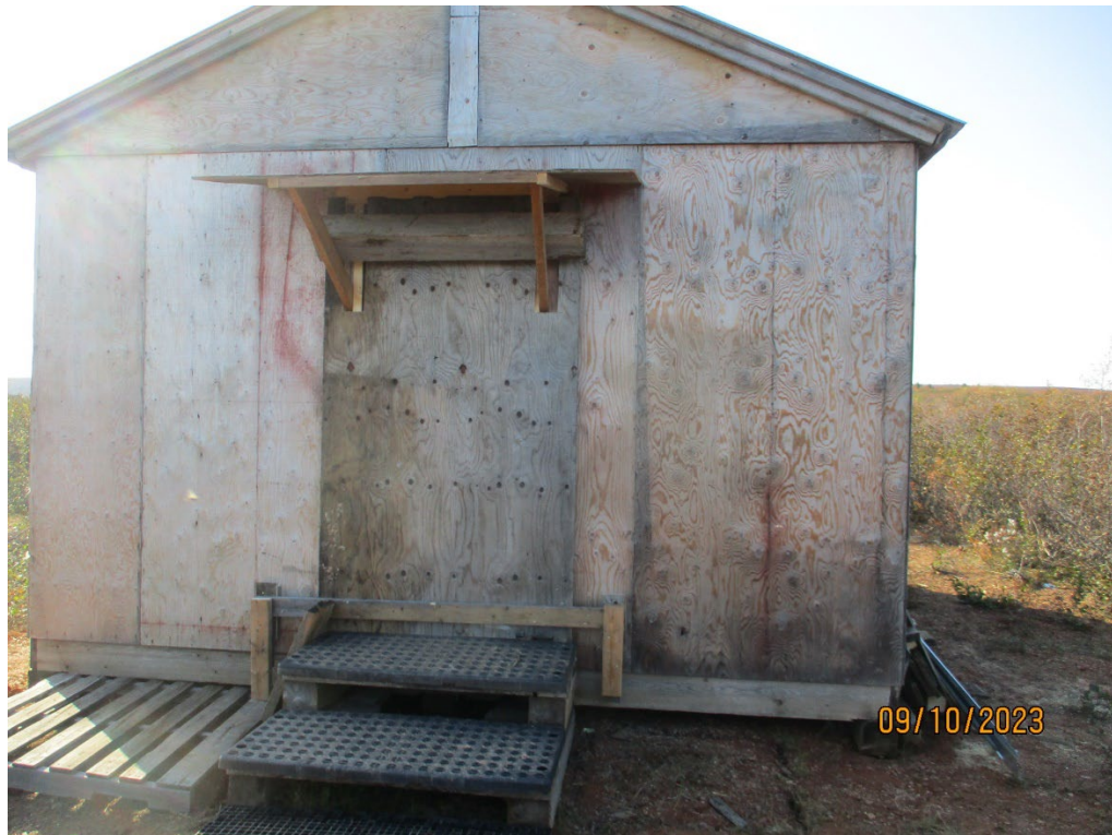
Photo 22: New survival shelter condition on leaving the site.
