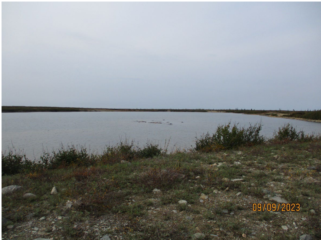
Photo 12: Tailings Pond No .1 waste rock island due to low water level.
