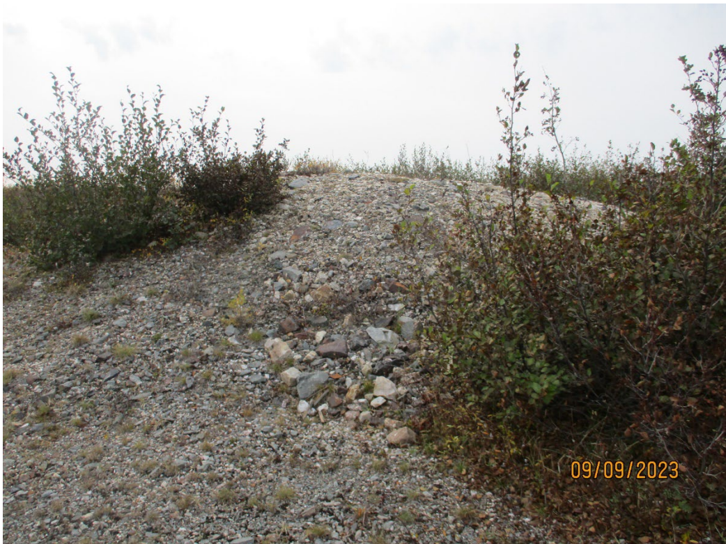
Photo 16: B-Zone raise fill mound.
