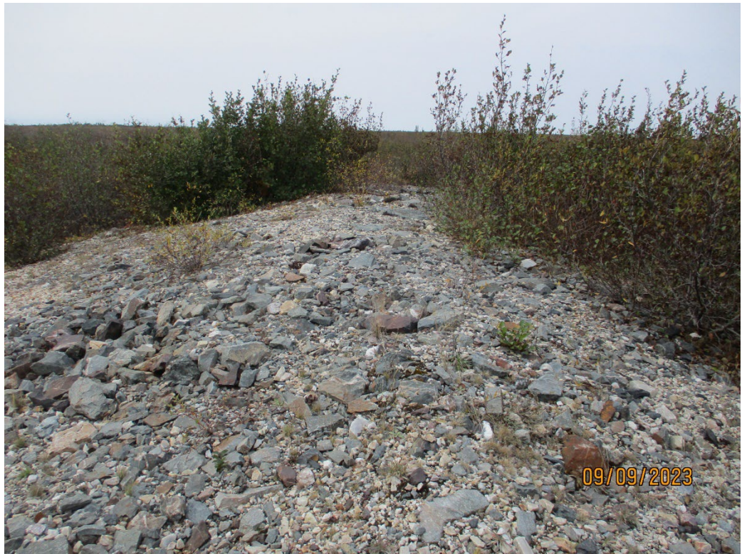
Photo 15: B-Zone Portal fill mound looking east.
