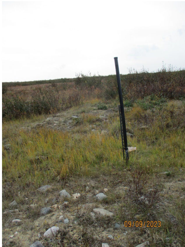
Photo 19: T3 thermistor casing intact.
