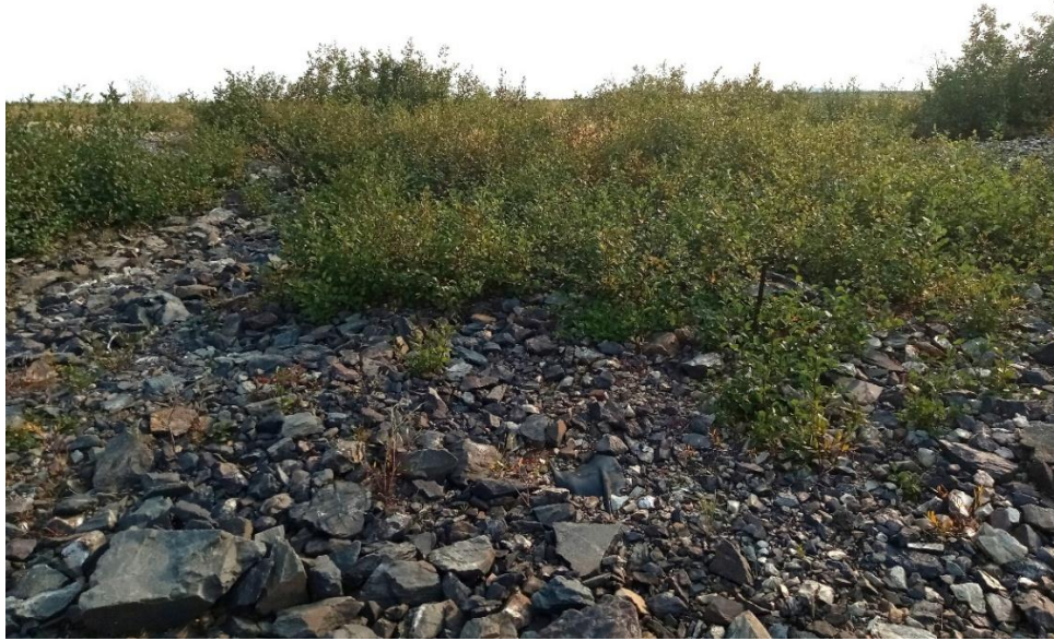
Photo 9: Tailings Pond No .1 spillway invert looking east.
