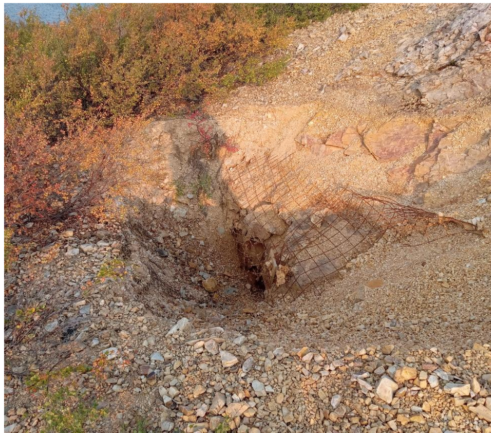
Photo 2: Shear Lake Portal subsidence at brow.
