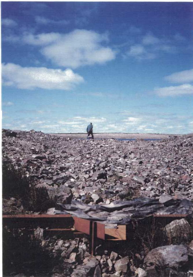
Photo 4. Spillway No. 1 looking upstream (west). Note flow measurement weir.
