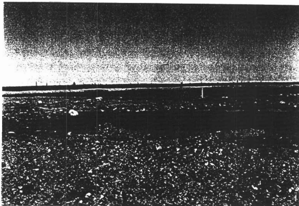
Figure 3: Surface depression in B-zone covered tailings area.
