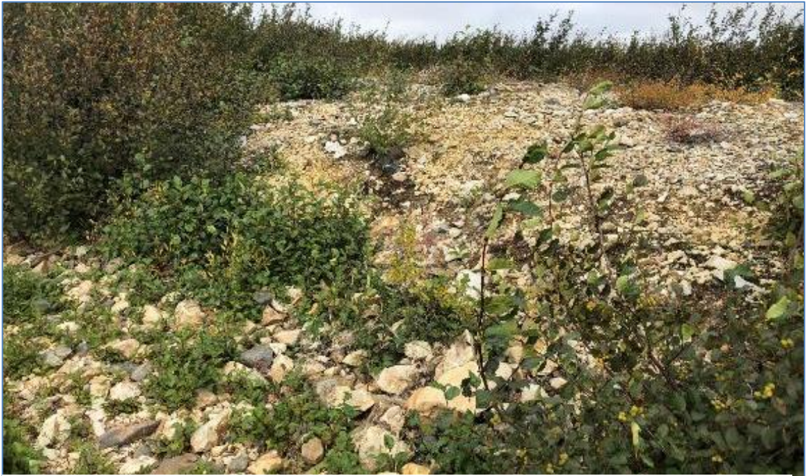
Photo 11: Minor sloughing on the upstream slope south of the low point.
