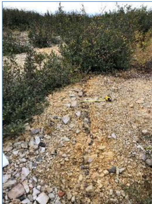
Photo 12: Longitudinal cracking self-armouring with rock and vegetation.
