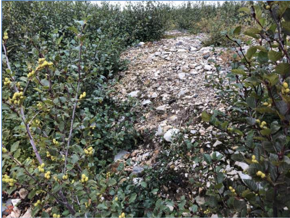
Photo 11: Minor sloughing on the upstream slope south of the low point.
