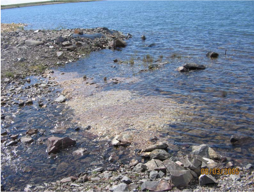
Photo 7: Dam No. 1 Spillway showing new fill at channel entrance
