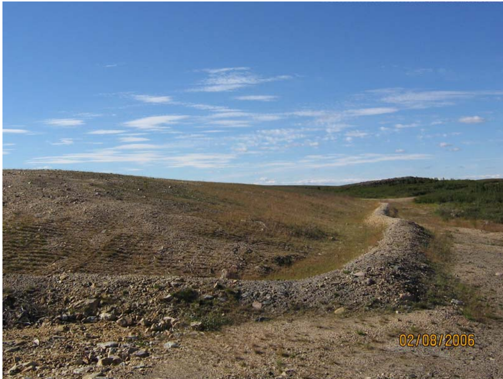
Photo 15: Looking north from southeast corner of Shear Lake Waste Rock Pile
