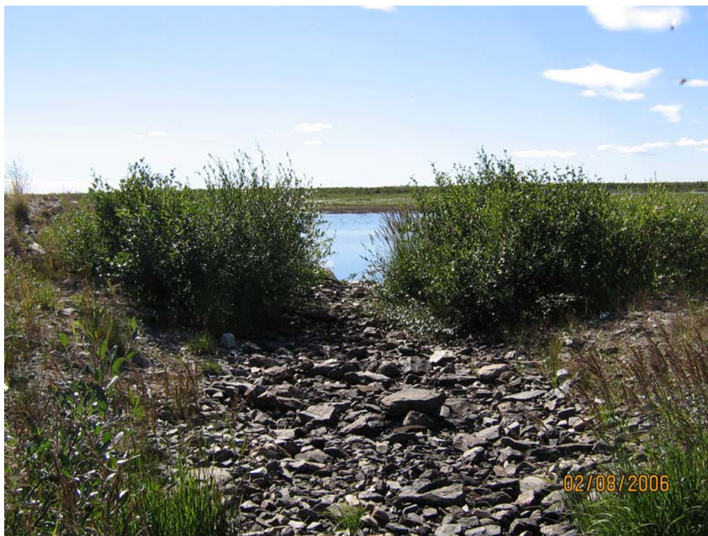
Photo 10: Dam No. 2 spillway looking upstream – note no flow
