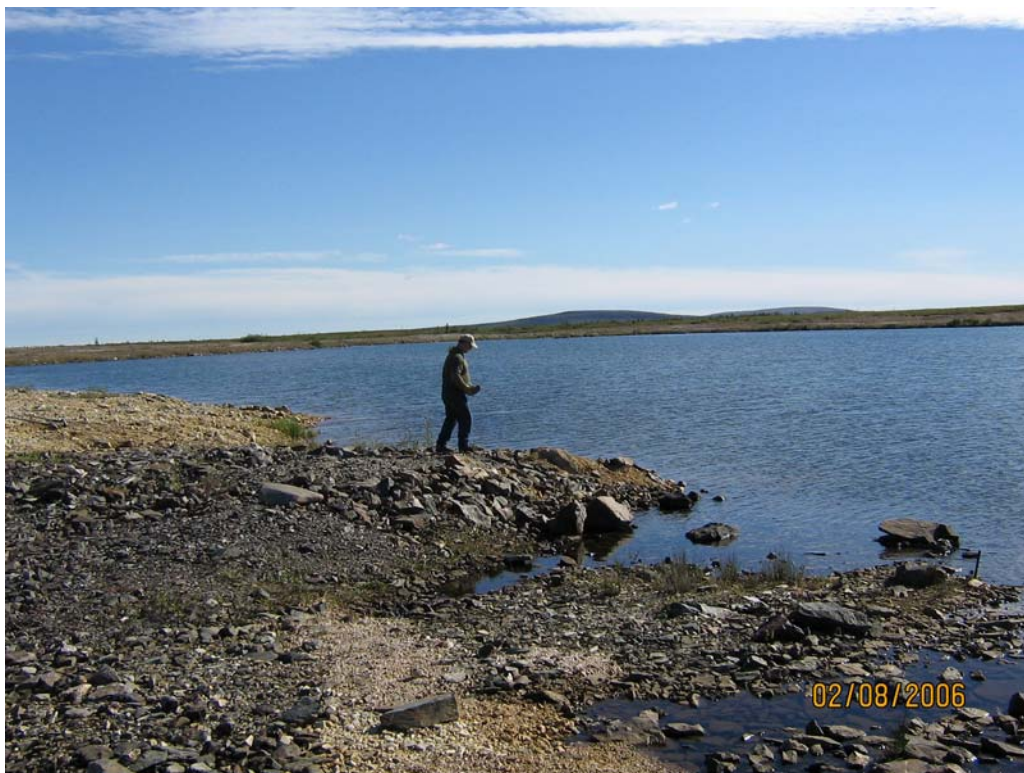
Photo 7: Dam No. 1 spillway south flank showing repairs below person
