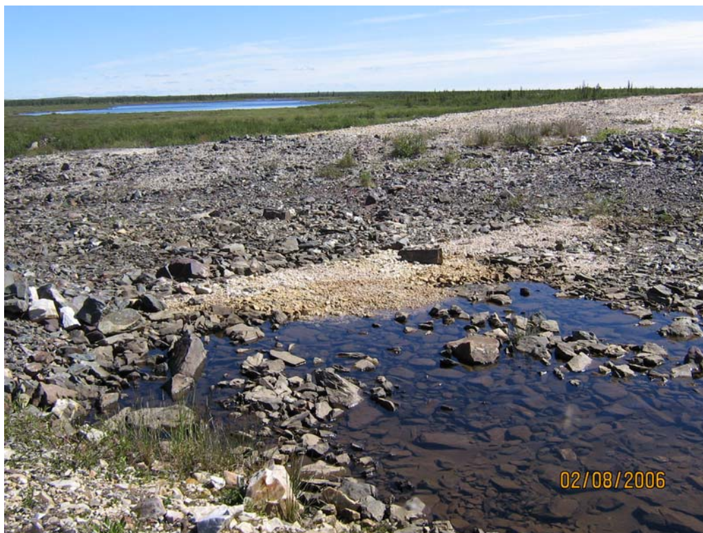
Photo 5: Dam No. 1 spillway looking downstream (no flow)
