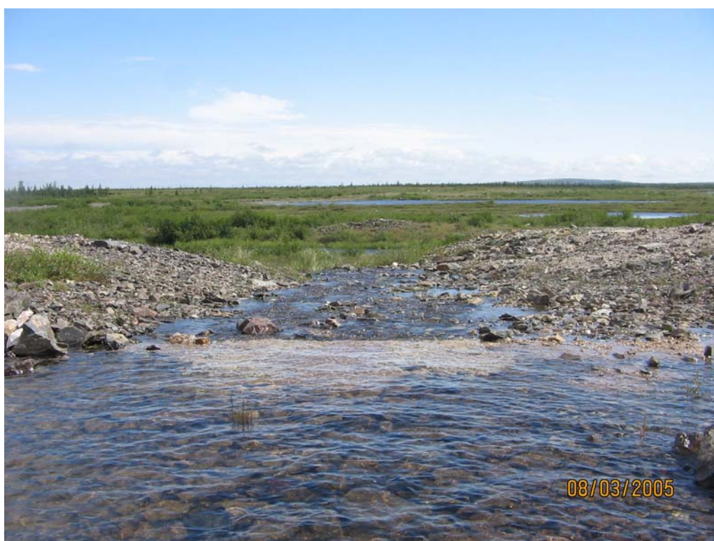
Photo 6: Dam No. 1 Spillway looking downstream (2005)
