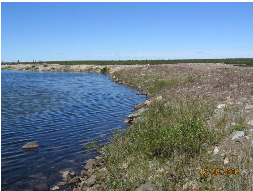
Photo 3: Dam No. 1 - looking northwest
