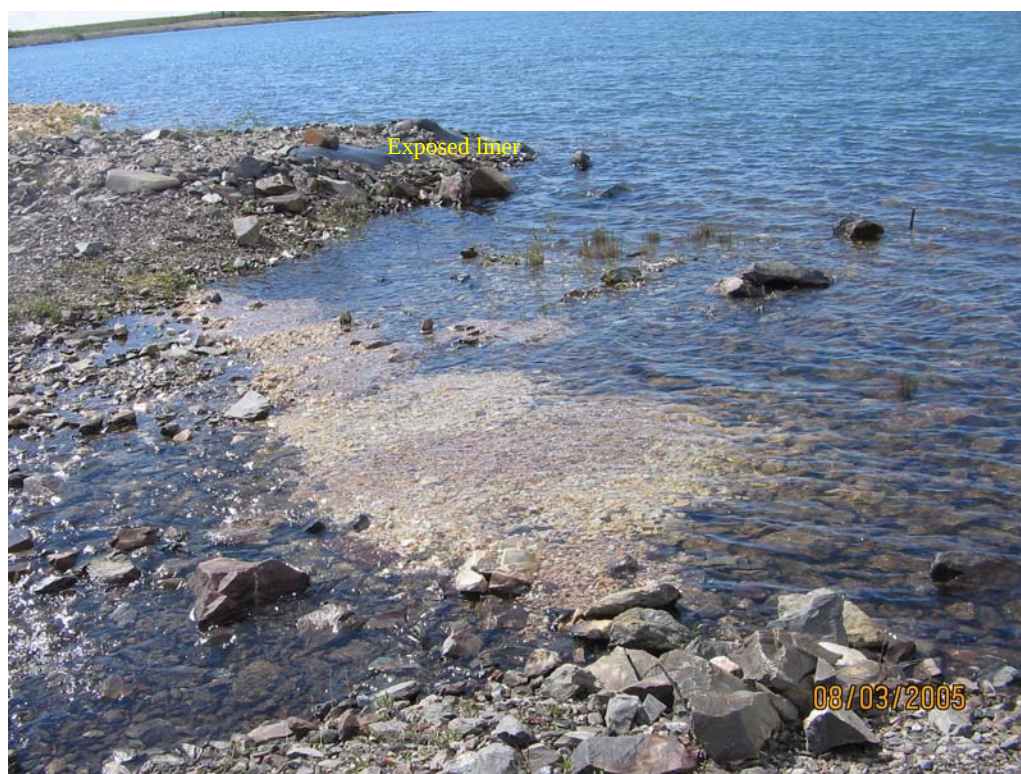
Photo 8: Dam No. 1 spillway entrance showing exposed rubber liner (2005)
