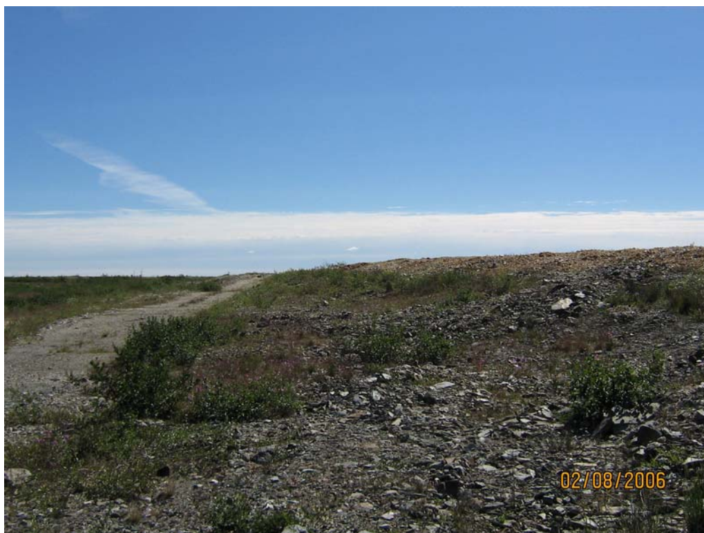
Photo 4: Downstream section of Dam No. 1
