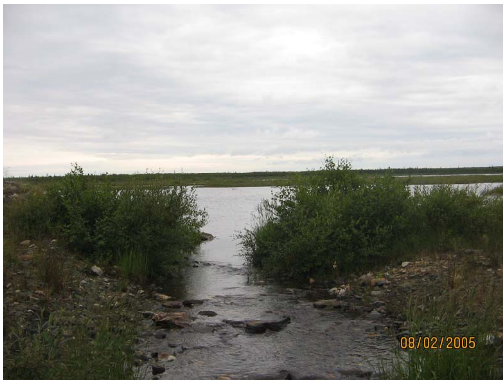
Photo 11: Dam No. 2 spillway looking upstream to Pond No. 2 (2005)
