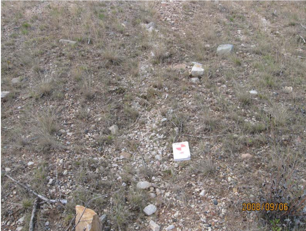
Photo 11: Previously gravel filled erosion channels on Shear Lake Waste Rock Pile
