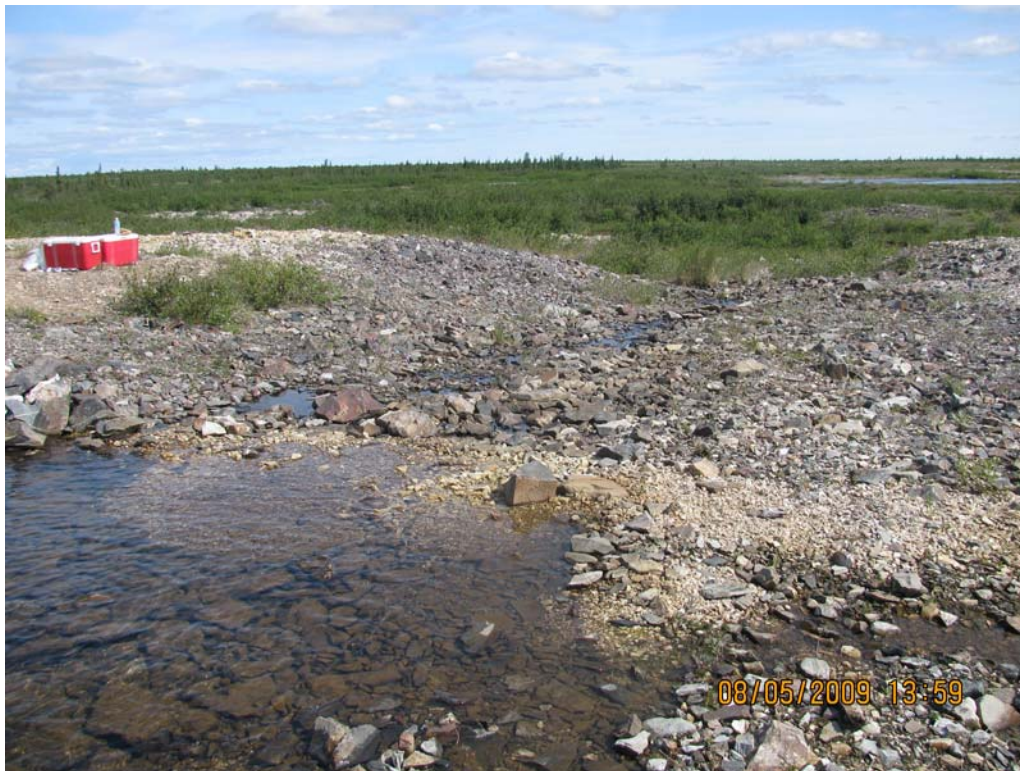
Photo 5: Dam No. 1 Spillway inlet looking downstream
