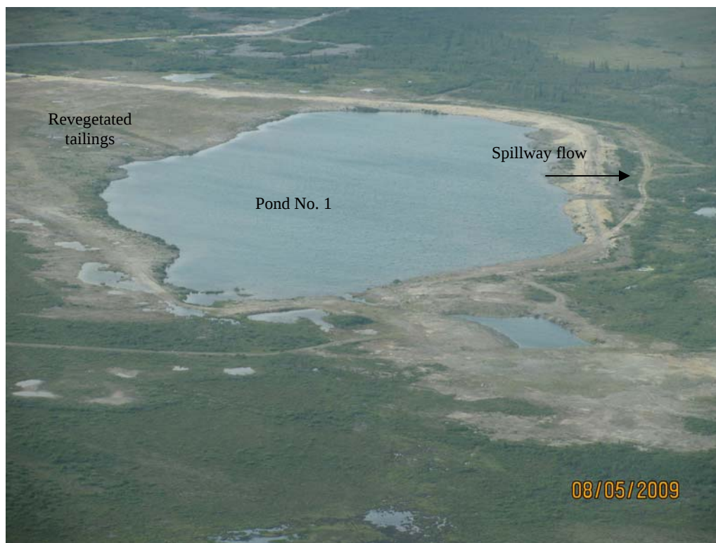
Photo 2: Tailings facility looking roughly northwest
