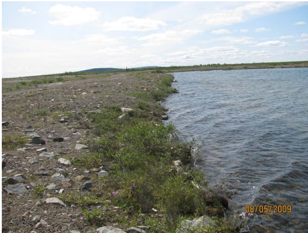
Photo 3: Dam No. 1 - looking south - southeast
