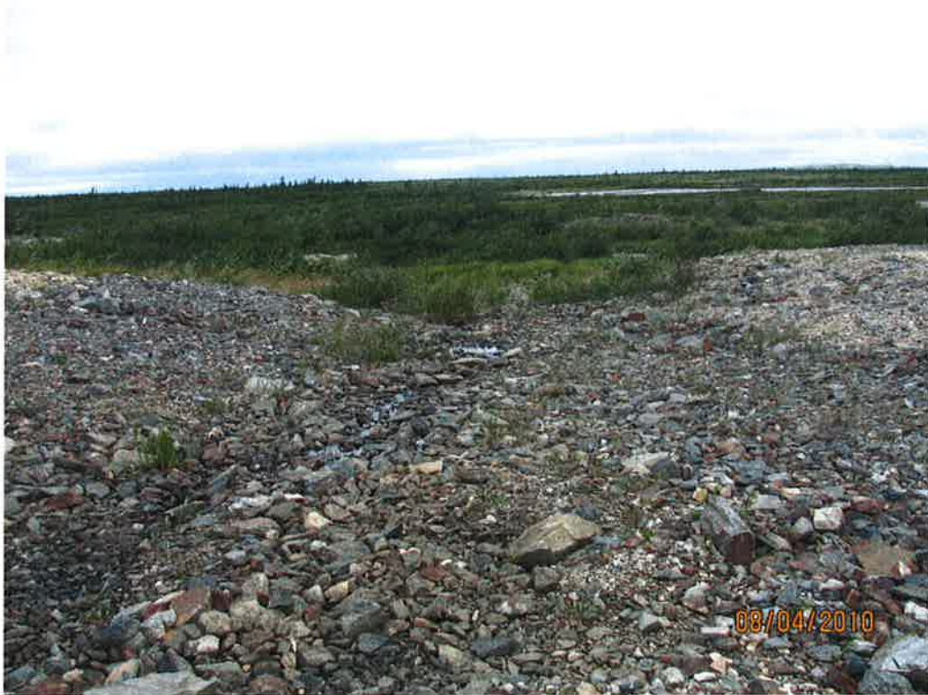
Photo 7: Dam No. 1 Spillway downslope channel
