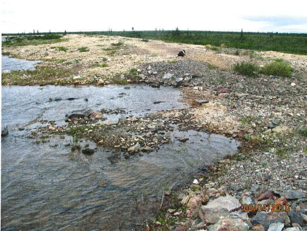
Photo 6: Dam No. 1 Spillway inlet and crest
