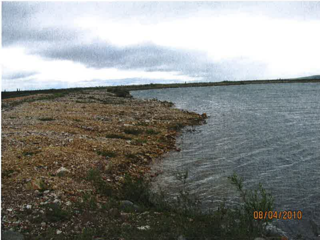
Photo 3: Dam No. 1 - looking south - southeast
