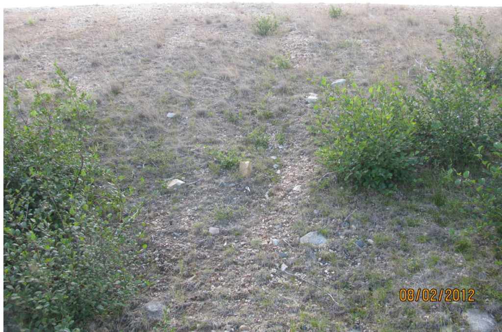
Photo 12: Previously gravel filled erosion channels on Shear Lake Waste Rock Pile
