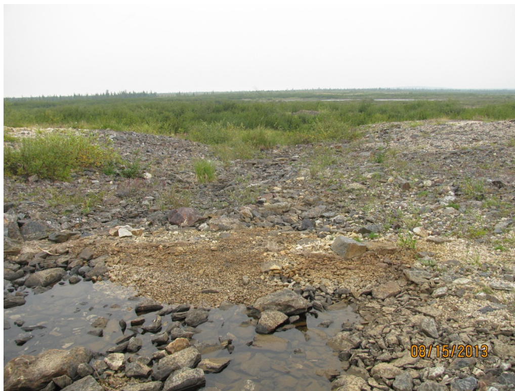
Photo 7: Dam No. 1 Spillway downslope channel
