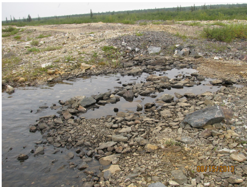
Photo 6: Dam No. 1 Spillway inlet and crest
