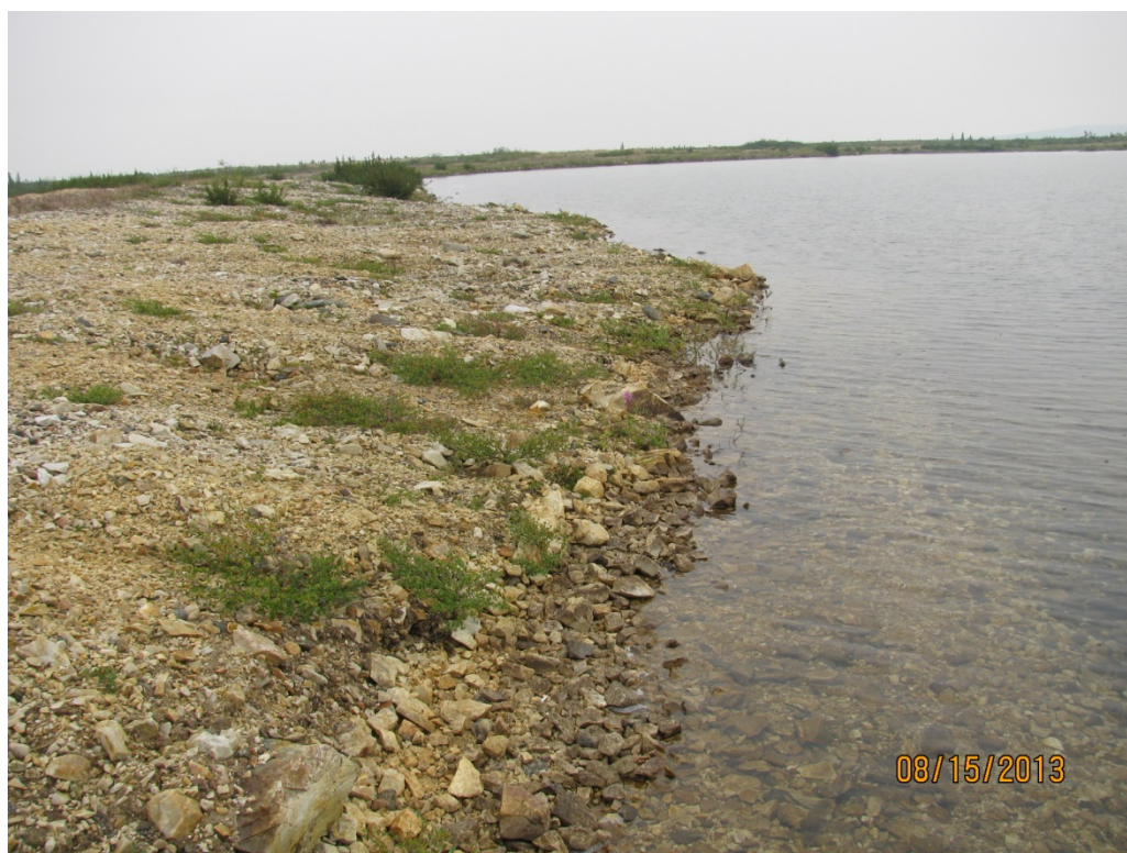
Photo 3: Dam No. 1 - looking south - southeast
