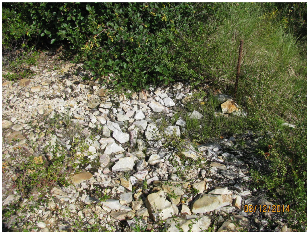
Photo 5: Wet spot on downstream side of Dam No. 1- no seepage
