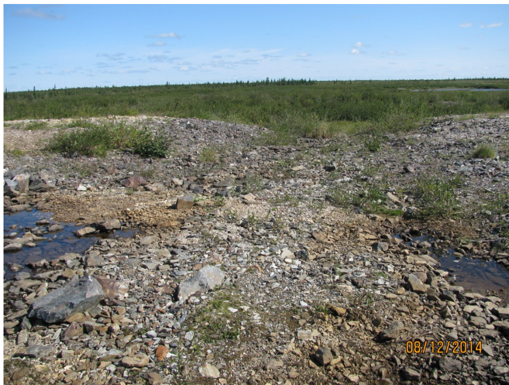
Photo 7: Dam No. 1 Spillway downslope channel
