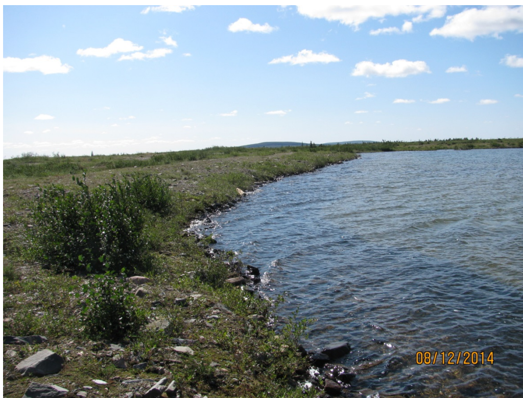
Photo 3: Dam No. 1 – upstream bank looking south
