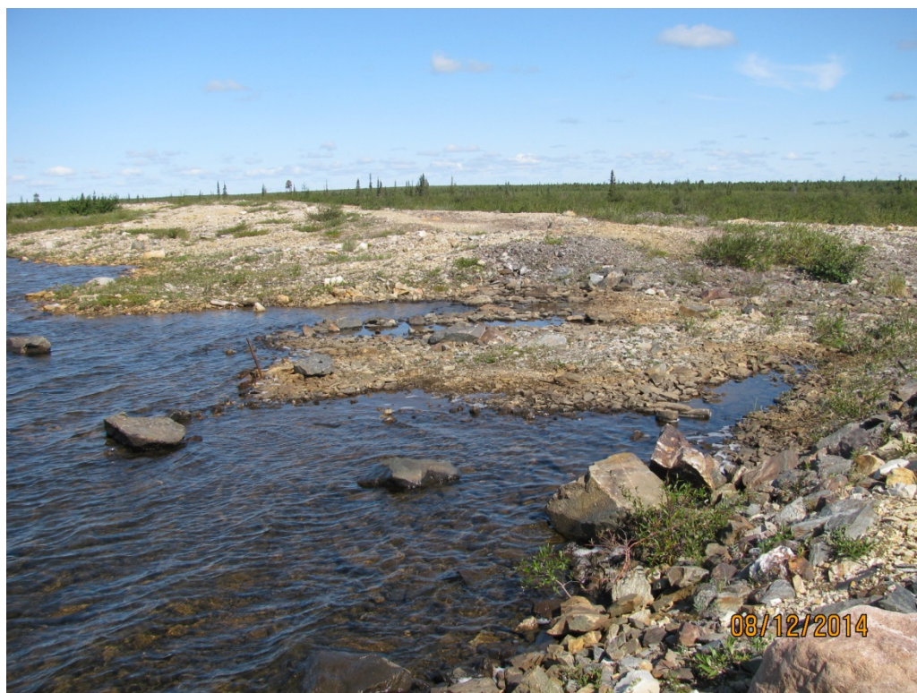
Photo 6: Dam No. 1 Spillway inlet and crest
