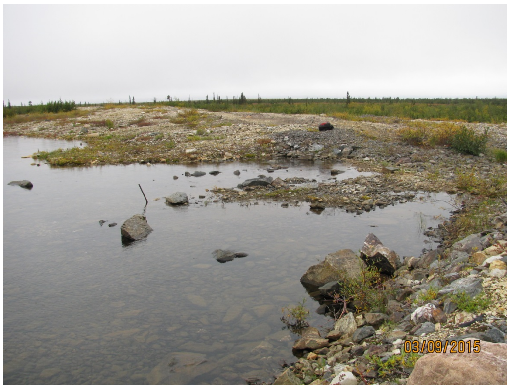
Photo 6: Dam No. 1 Spillway inlet and crest
