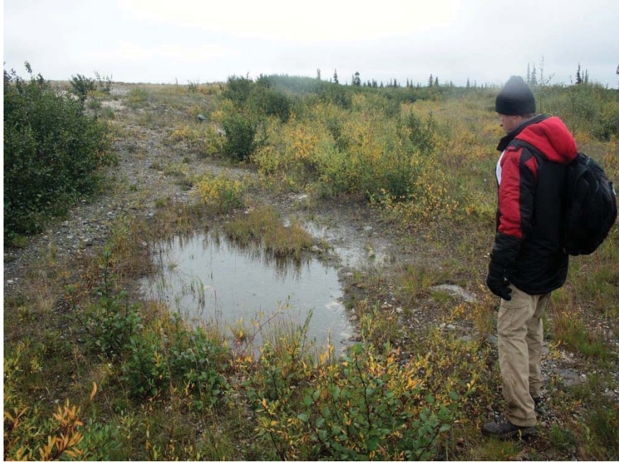
Photo 11. Wet patch on downstream toe of TP1 with D. Georgiou, P.Eng.
