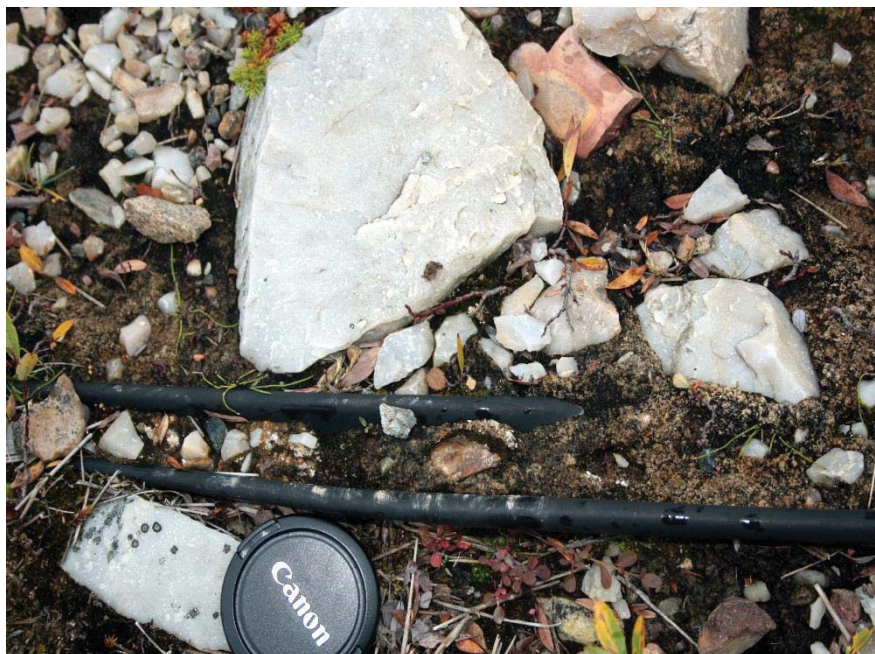
Photo 8. Exposure of edge of liner in spillway.
