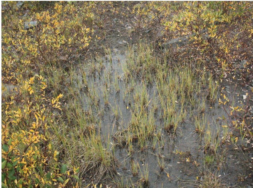
Photo 12. Semi-permanent wet area at downstream toe. (Ref D. Georgiou)
