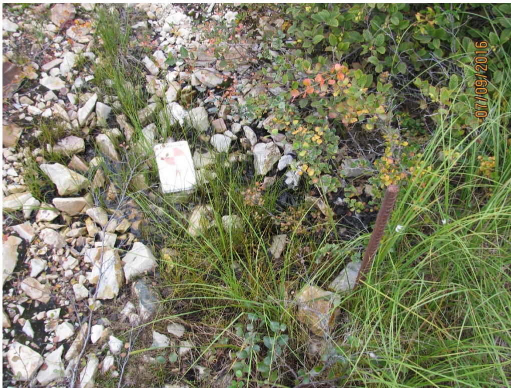
Photo 5: Wet spot on downstream side of Dam No. 1- minor seepage/ponding
