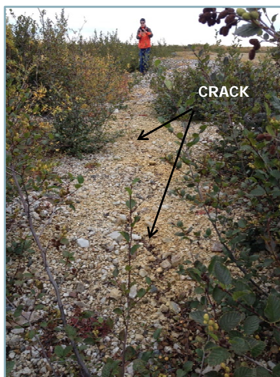
Photo 10: Cracking where access road adjoins Dam 1 crest (looking south).
