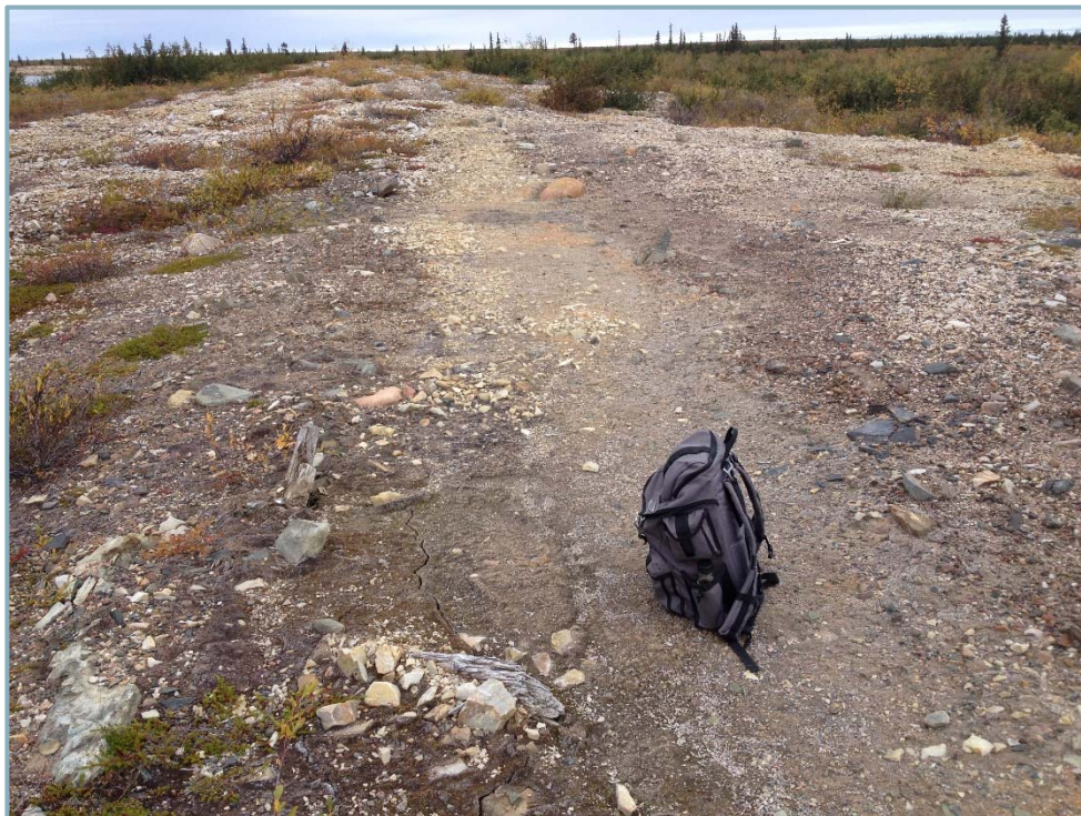
Photo 11: Localized surface cracking north of TP1 spillway (looking north).
