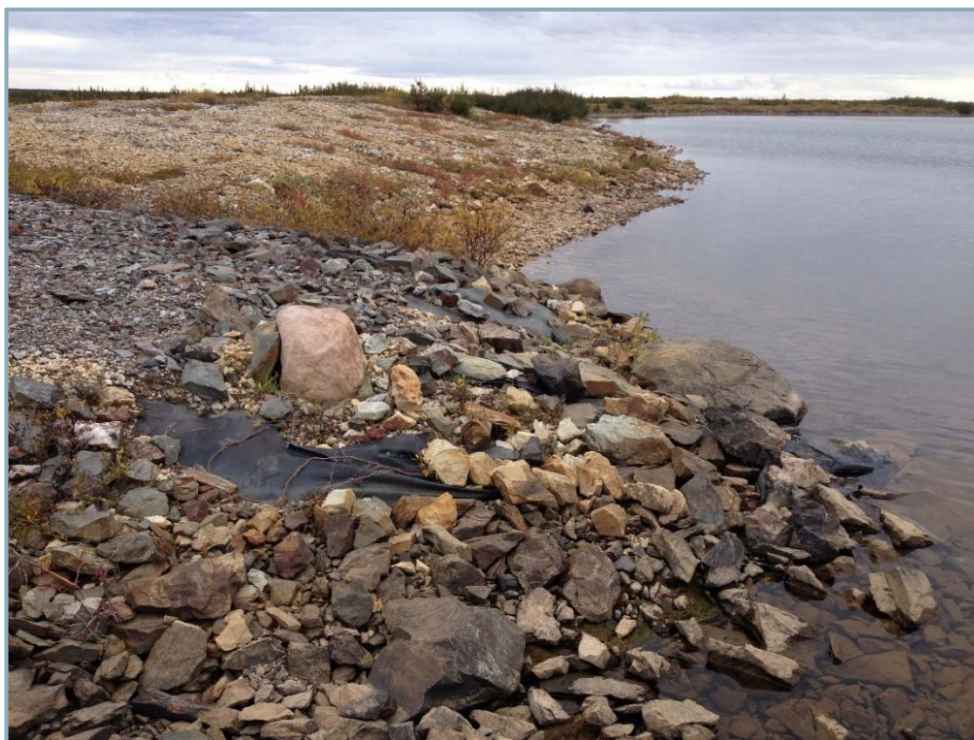
Photo 12: Liner exposed at the south edge of TP1 spillway (looking south).
