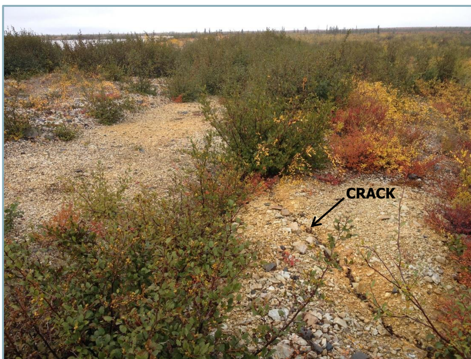
Photo 12: Cracking where access road adjoins Dam 1 crest (looking north).
