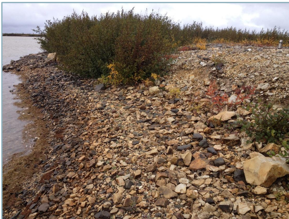
Photo 11: Minor sloughing on upstream slope (looking north).
