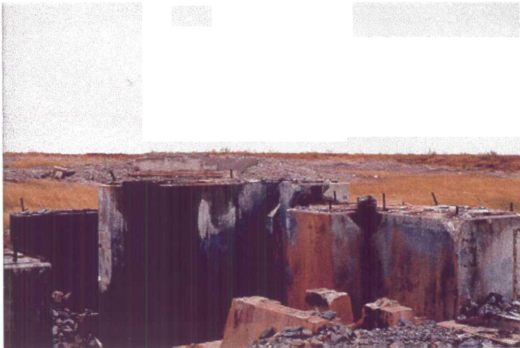
Foundations at mill site. The exposed rebar will be removed.
