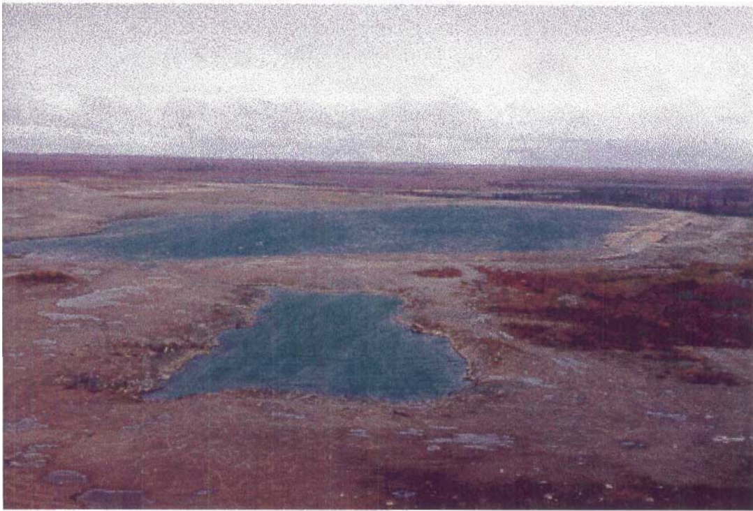
Quarry pit in foreground with tailings pond behind. The quarry and ditch connecting it to the tailings pond have filled with water.
