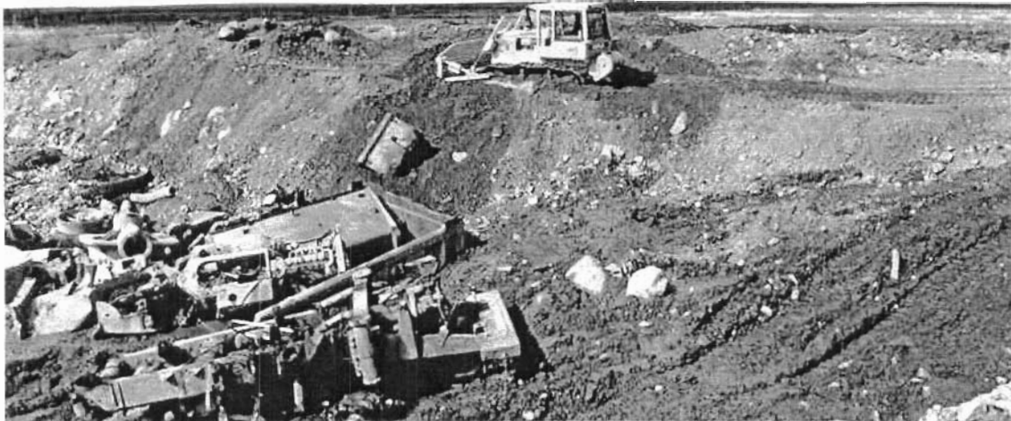
Cover being placed on Quarry Pit
