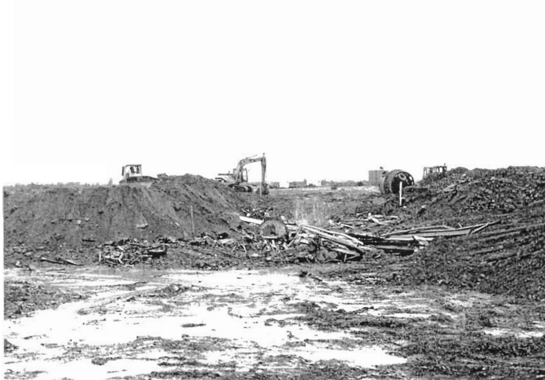
Dozer and Hoe flattening scrap material
