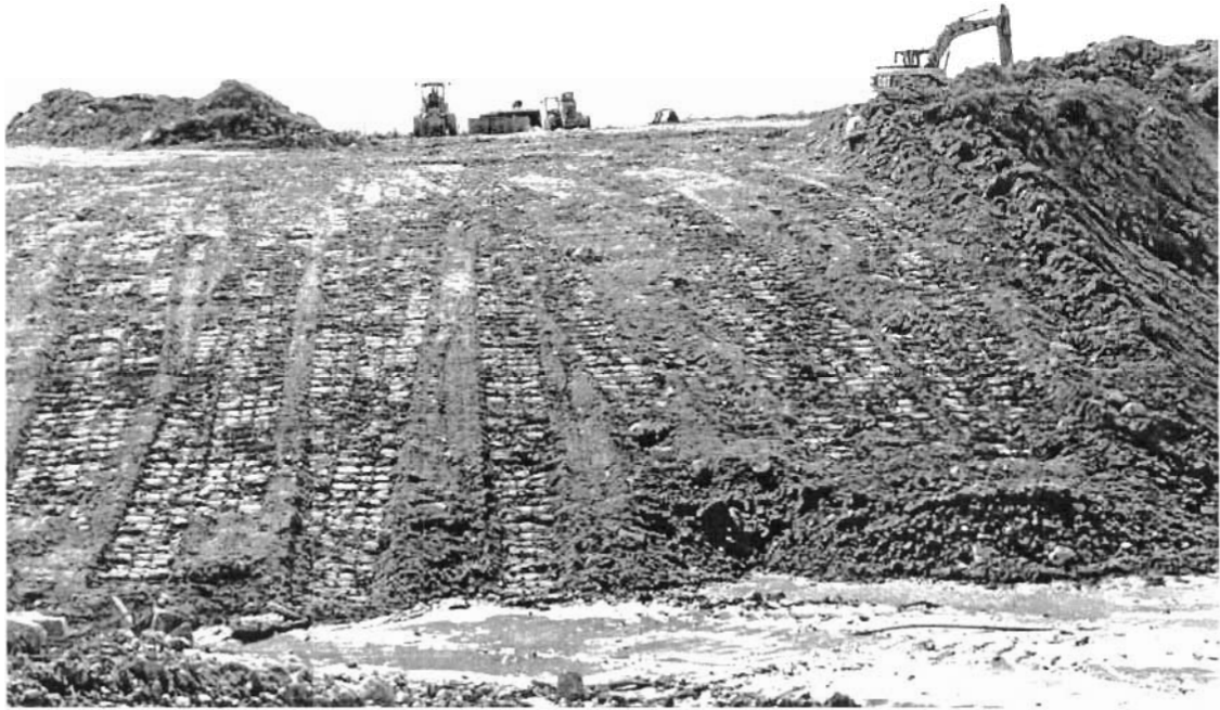
Final slope on Quarry Pit Cover
