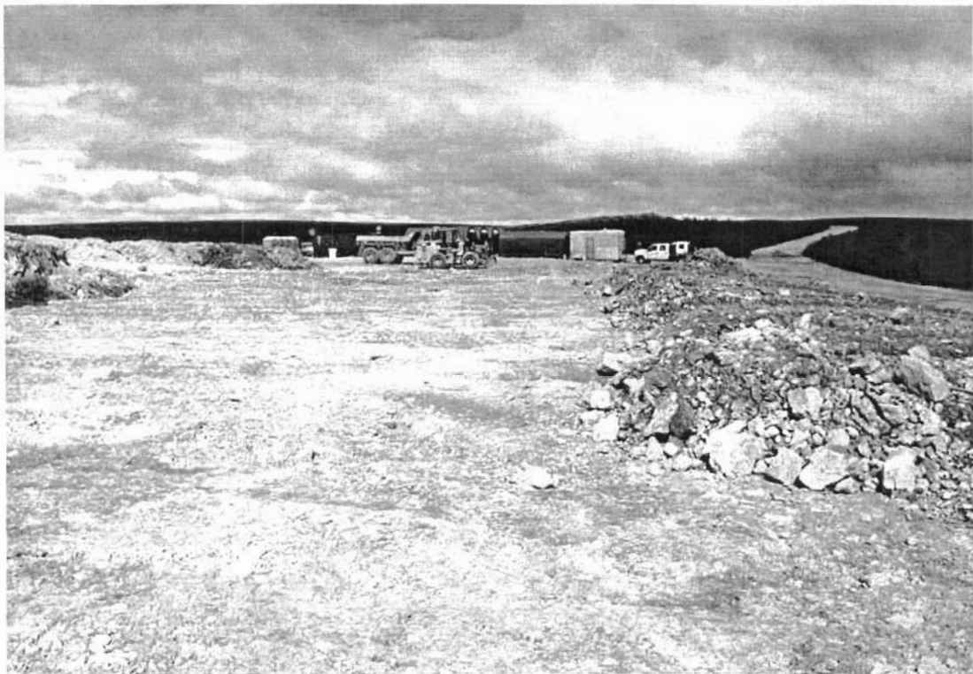
Base prepared for waste rock encapsulation
