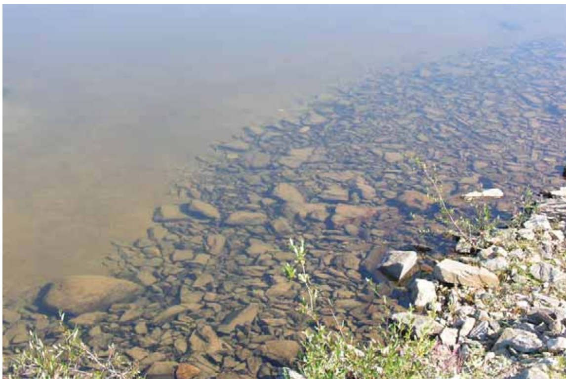
Figure 3-1: Subaqueous Boundary Between Uncovered Tailings and Cover Apron
