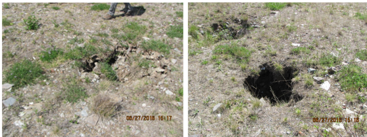
Photograph 5-13. Settlement areas in southeast corner of quarry pit cover (left) and new sinkholes identified in 2016 (right).
