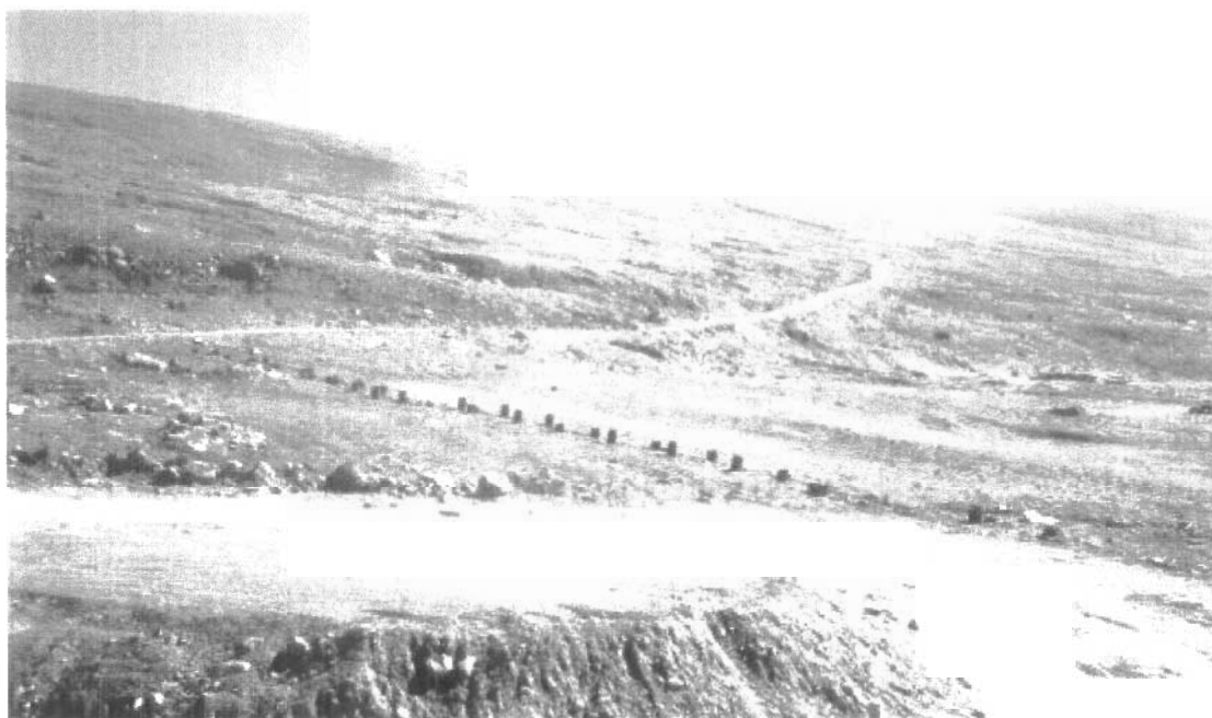
Photo 2 – Barrels mark POL Line from beach to Upper Site
