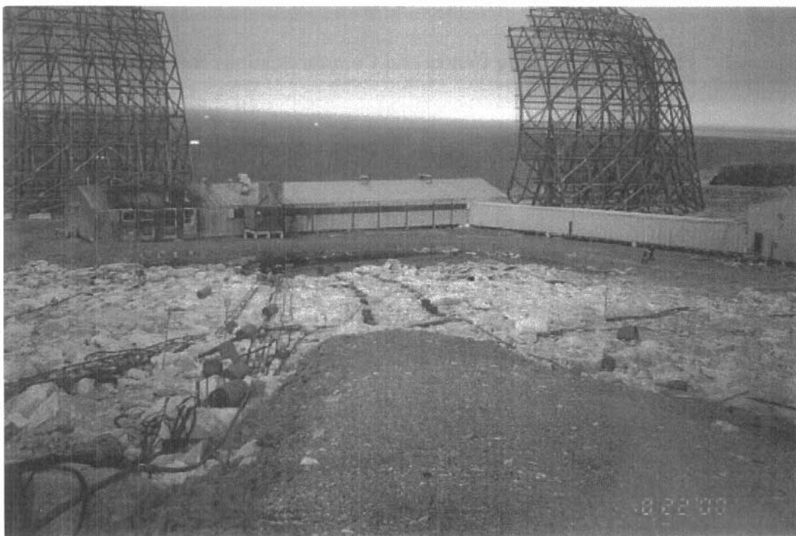
Photo 26 – DEW Drop Area including Communication and Power Cables
