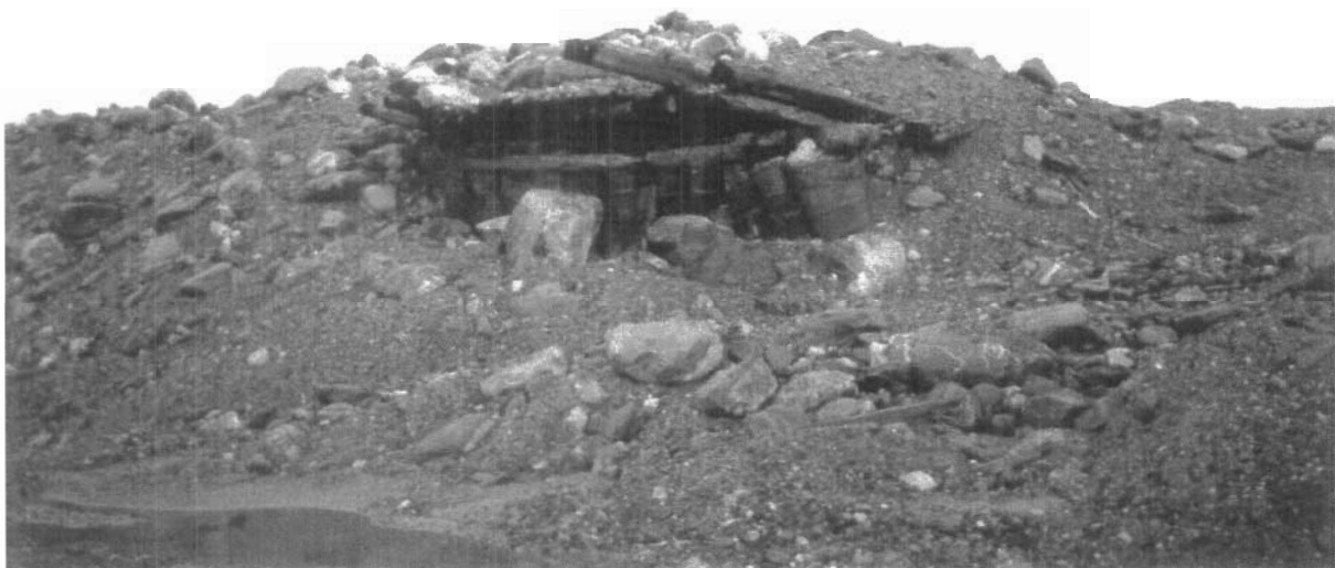
Photo 2 – Debris Area No. 63 (Dwg. 101)
