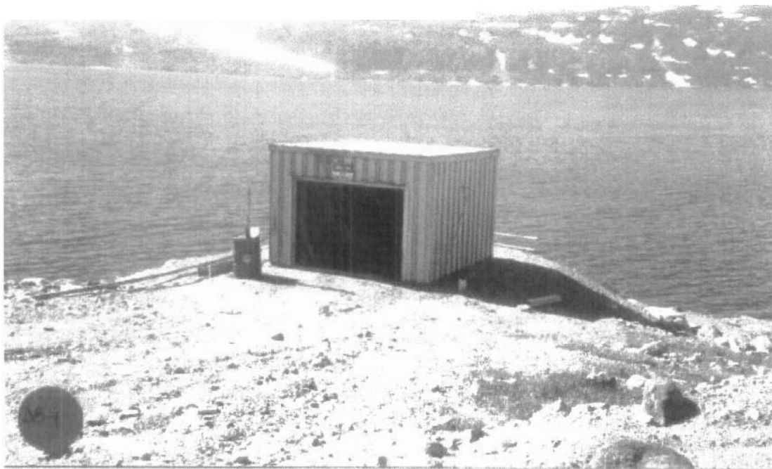
Photo 1 – Beach Area Pump House
