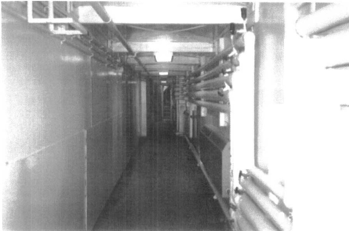
Photo 17 – Overhead Walkway Interior
