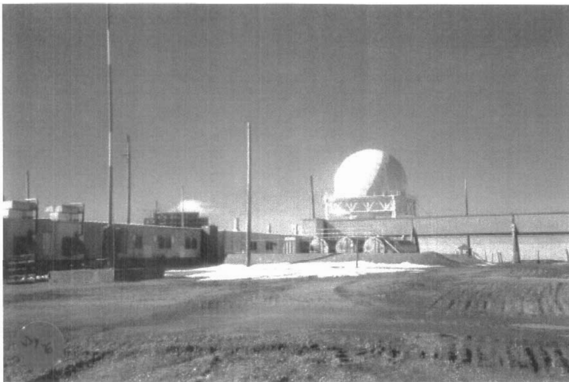
Photo 13 – Fuel Tank and Wood Antenna Poles
