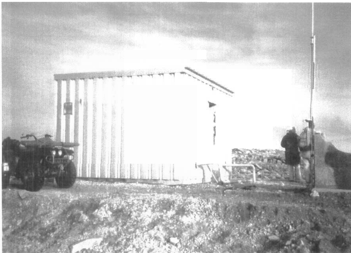
Photo 9 – Middle Site Valve Manifold House and Tank Support Structure
