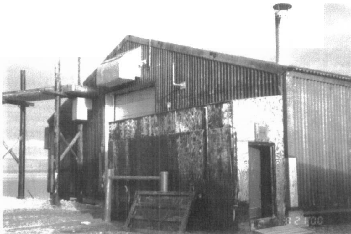
Photo 10 – Radio Terminal Building and C.E. Maintenance Shop
