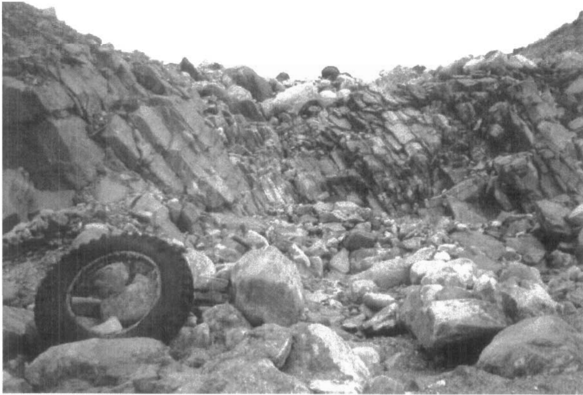
Photo 33 – Debris Area No. 19 (Dwg. 105)
