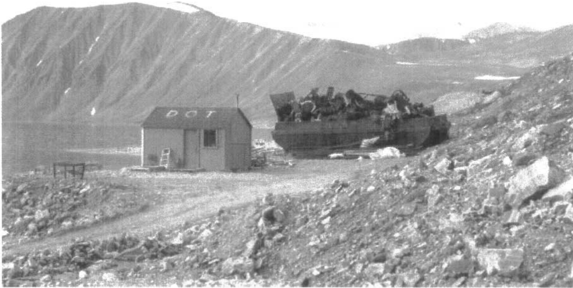
Photo 21 – Debris Area No. 16 (Dwg. 104)
