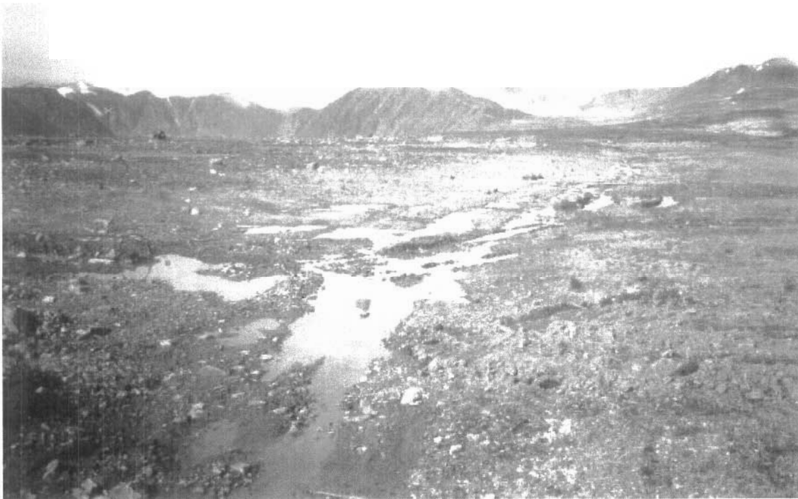
Photo 42 – Debris Area and Powerhouse Landfill (Dwg. 108)
