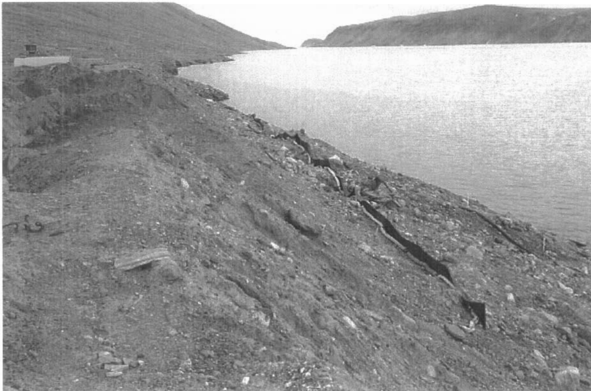
Photo 22 – Debris Area No. 17 (Dwg. 104)
