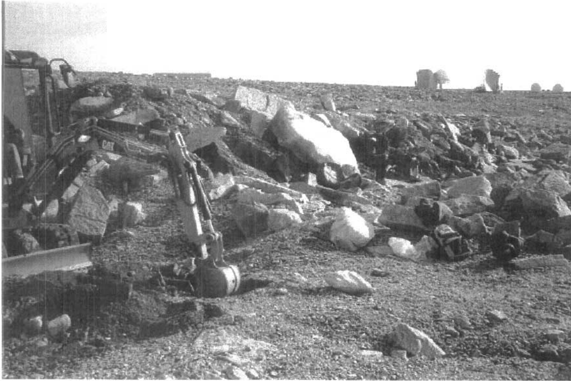
Photo 97 – Pallet Line Landfill (Dwg. 166)
