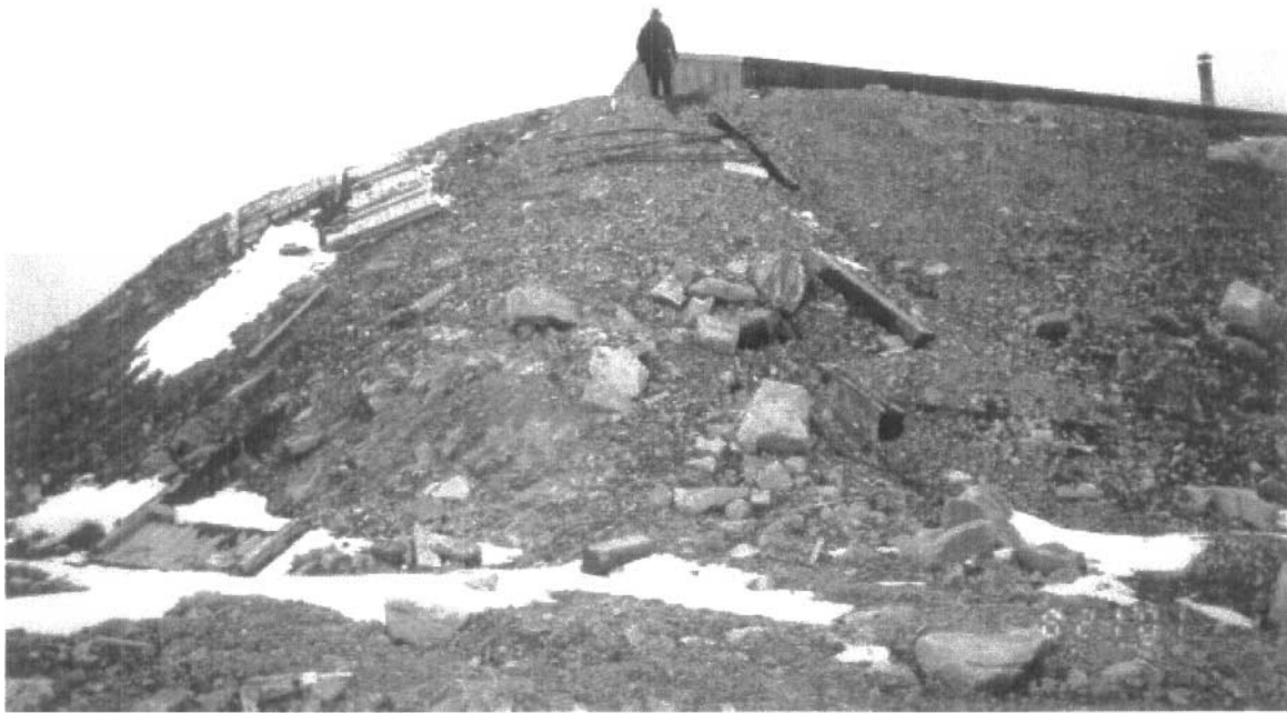
Photo 74 – Debris Area No. 48 (Dwg. 163)
