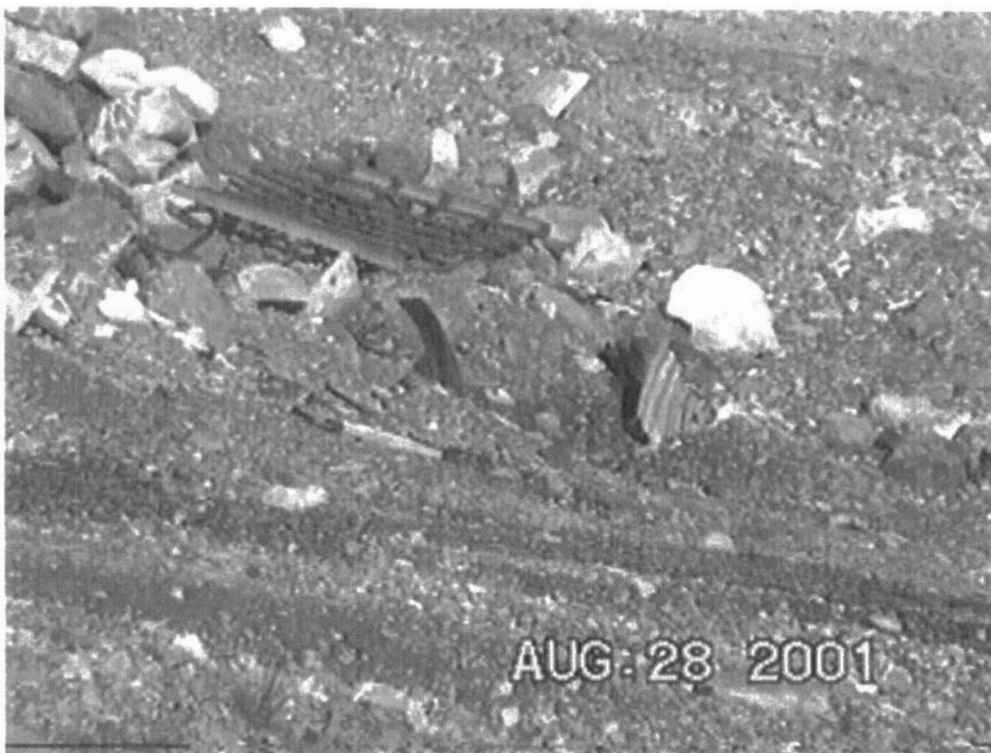
Photo 65 – Debris Area No. 38 (Dwg. 150)
