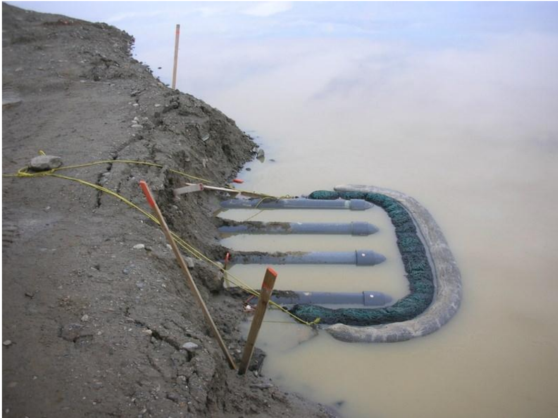
Figure 2. Photograph of oil-absorbent booms placed around intake of overflow pipes within landfarm.
