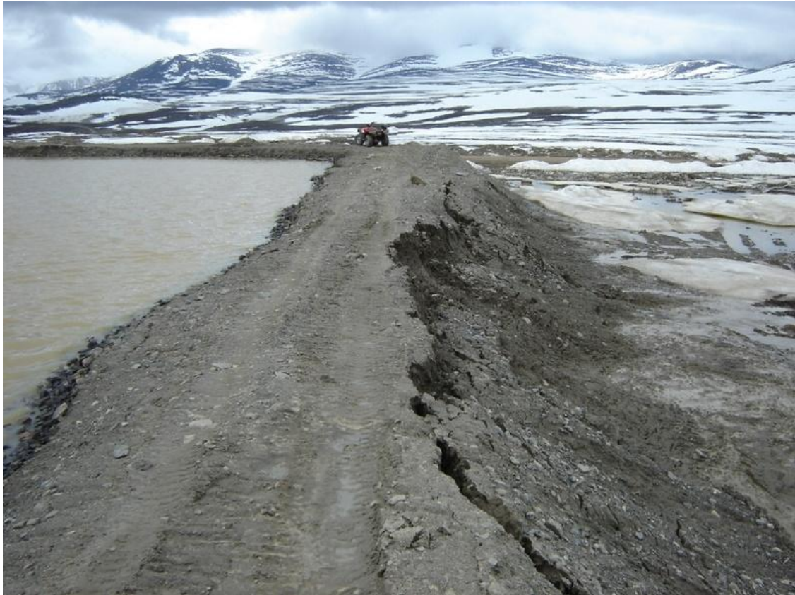
Figure 5. East berm of landfarm facility exhibiting cracking.
