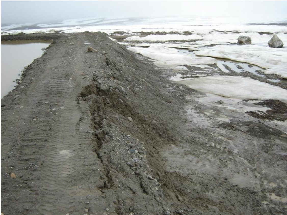
Figure 4. East berm of landfarm facility exhibiting sloughing on the outer side.
