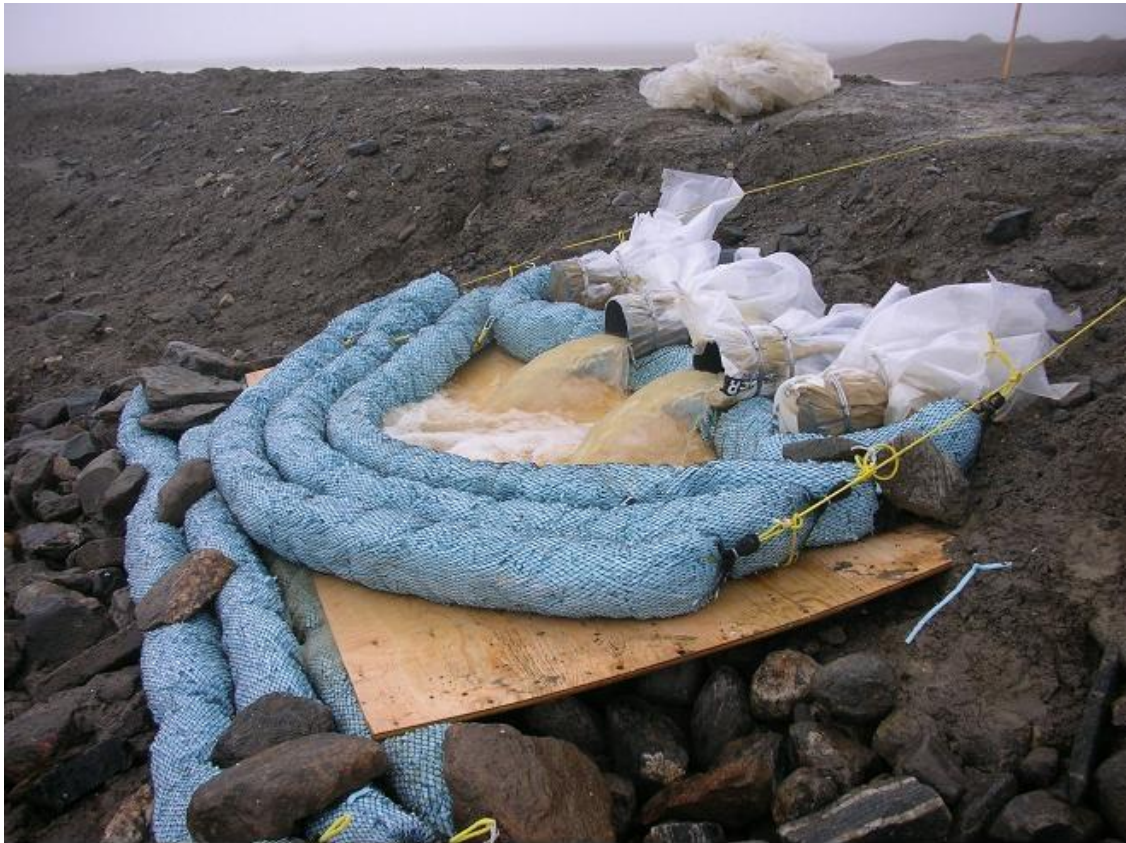
Figure 3. Photograph of oil-absorbent booms placed around discharge of the overflow pipes external to the landfarm.
