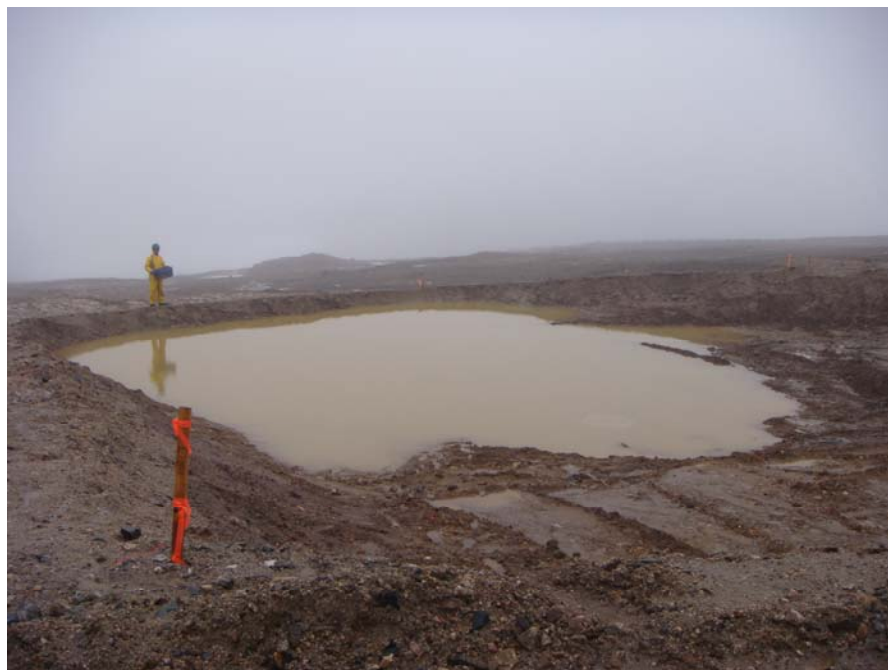
Photograph 26 (DSCO2985): West Landfill facing west, showing pooled wastewater at excavation base.
