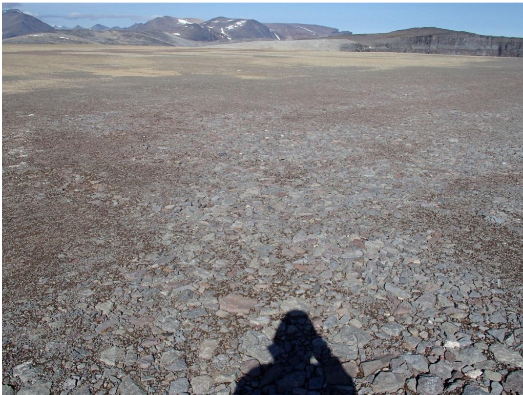
Photograph 31. Area of segregation on the southeast corner of the landfill ↑
