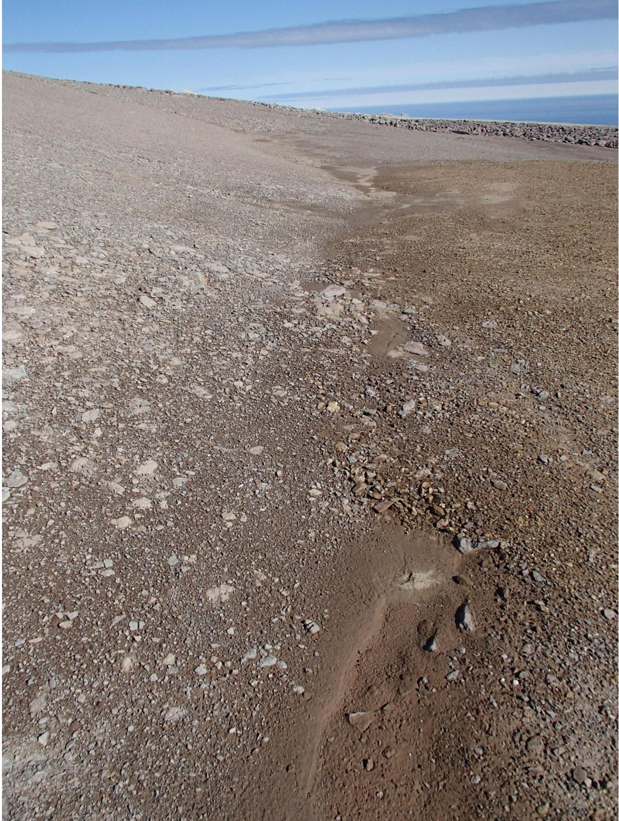
Photograph 50. Sedimentation along the ridge at the centre of the landfill ↑
