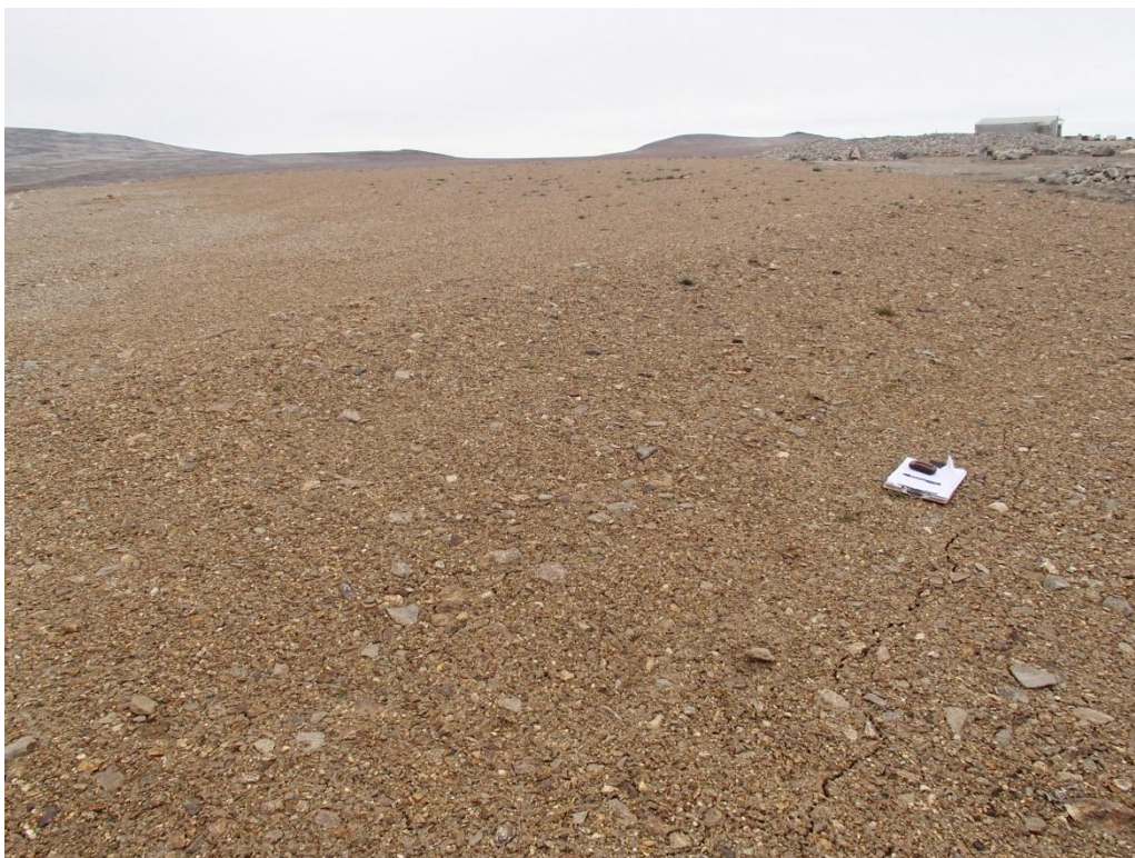
Photograph 91. Minor tension cracks in the landfill surface ↑
