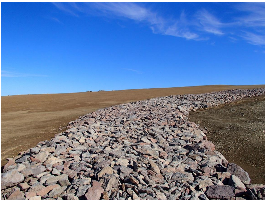
Photograph 23. Type 1 granular fill along the south toe ↑
