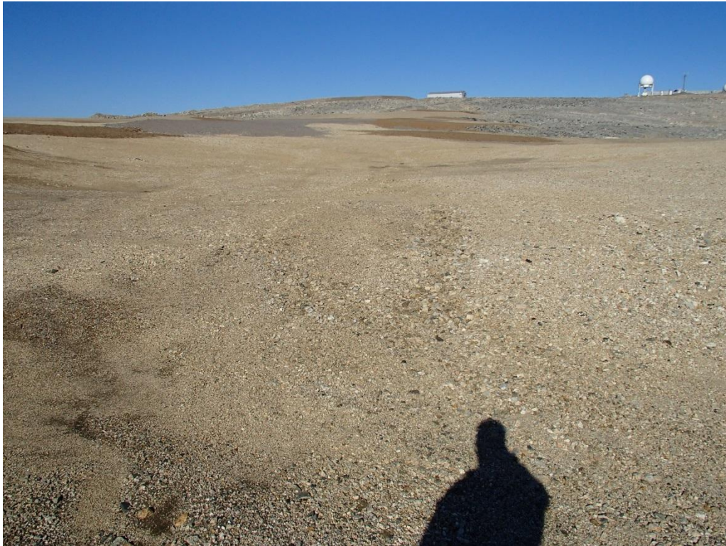
Photograph 76. Low area and area of minor erosion on Lobes 2, 3 and 4 ↑
