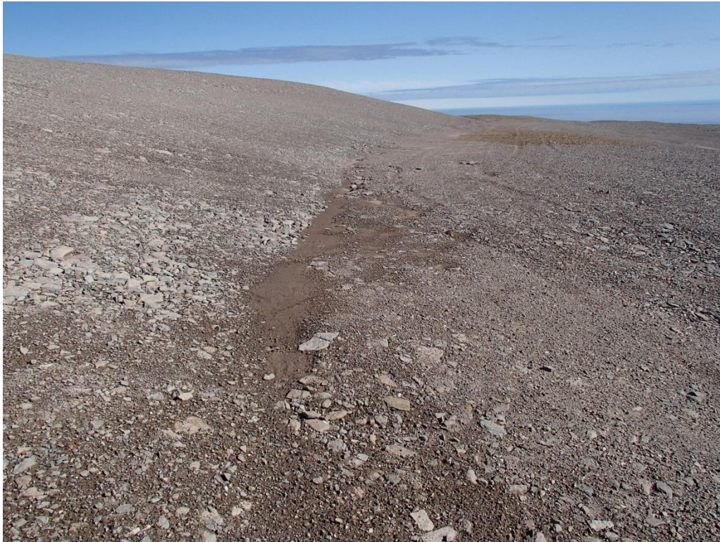
Photograph 51. Sedimentation along the ridge in the landfill ↑
