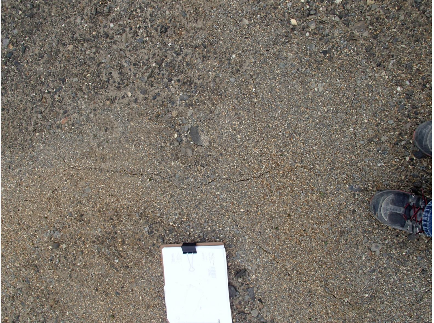
Photograph 85. Minor tension cracks in the landfill surface ↑
