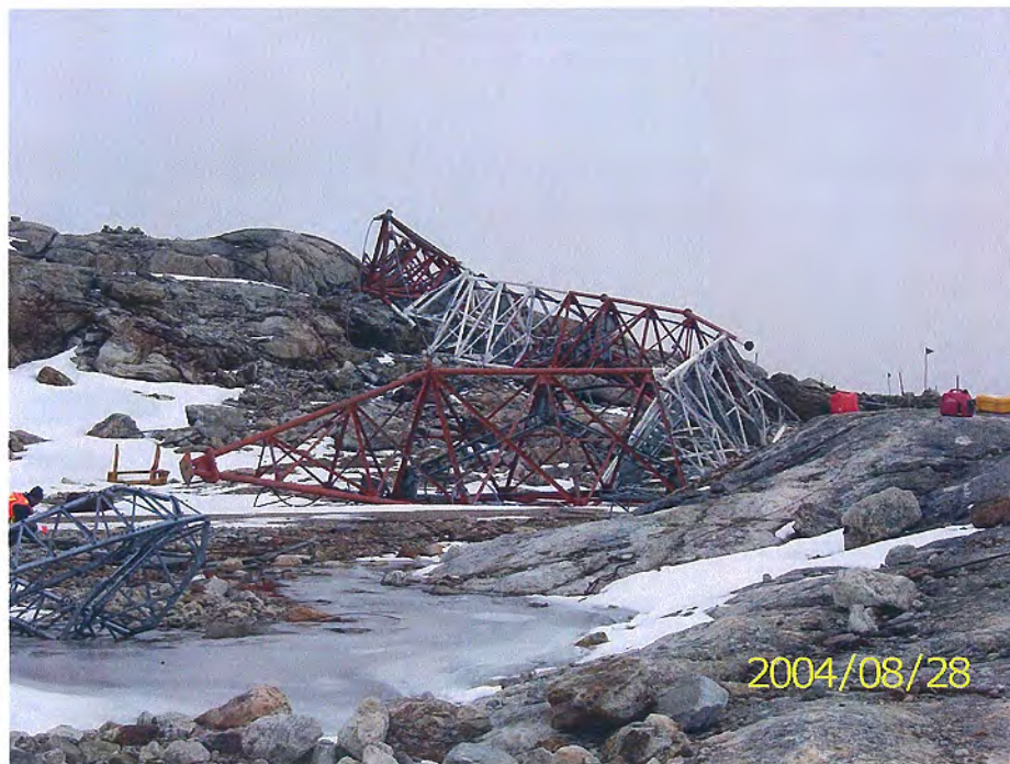
Photo 47 Downed antenna structure
