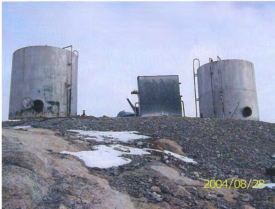
Photo 39 POL Storage Facility, looking north
