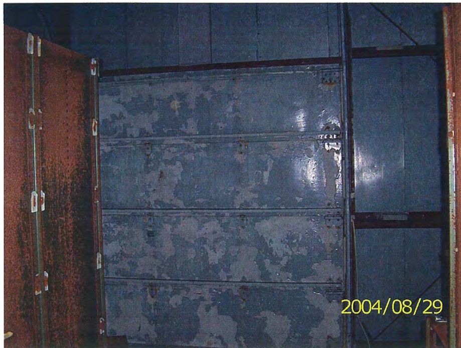
Photo 52 Overhead door and exterior wall cladding – Warehouse
