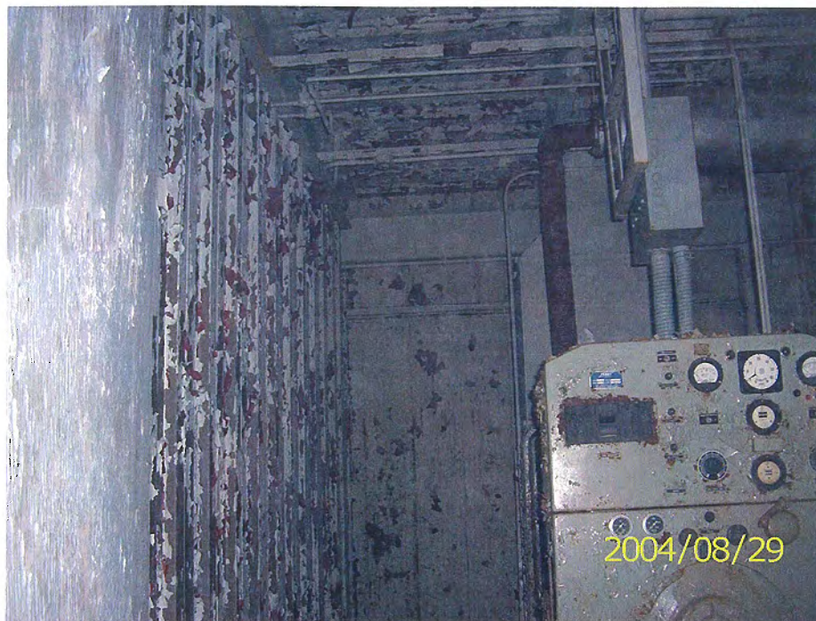
Photo 53 Genset and peeling paint in Generator Room – Garage
