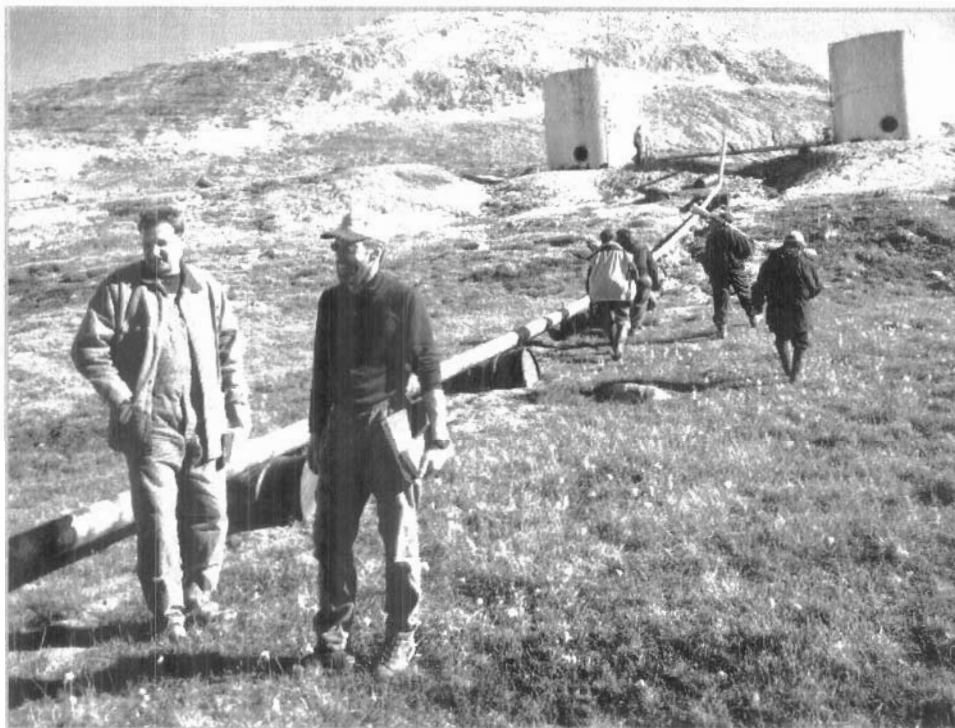
Photo 2 - Beach Area and POL Storage Tanks
