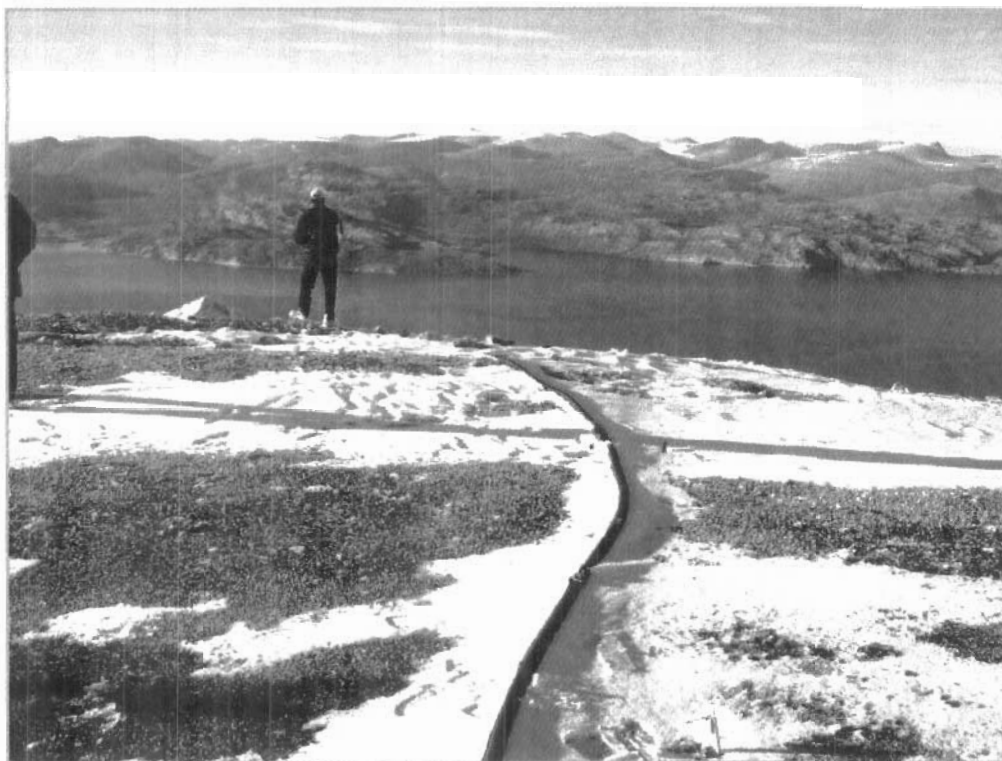
Photo 10 - Sewage Outfall from Module Train
