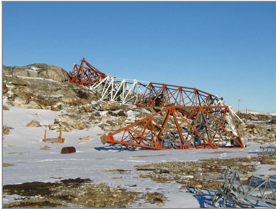
Photo 15 - Collapsed Antenna
