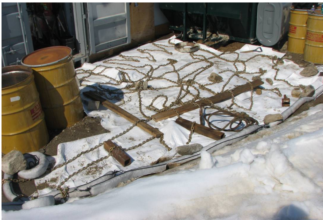
Figure 4 : Sorbent pads and booms around decontaminated area
