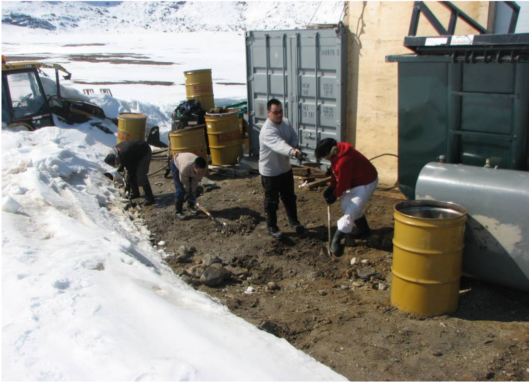
Figure 3 : Shovelling of contaminated soil into yellow Overpack Drums
