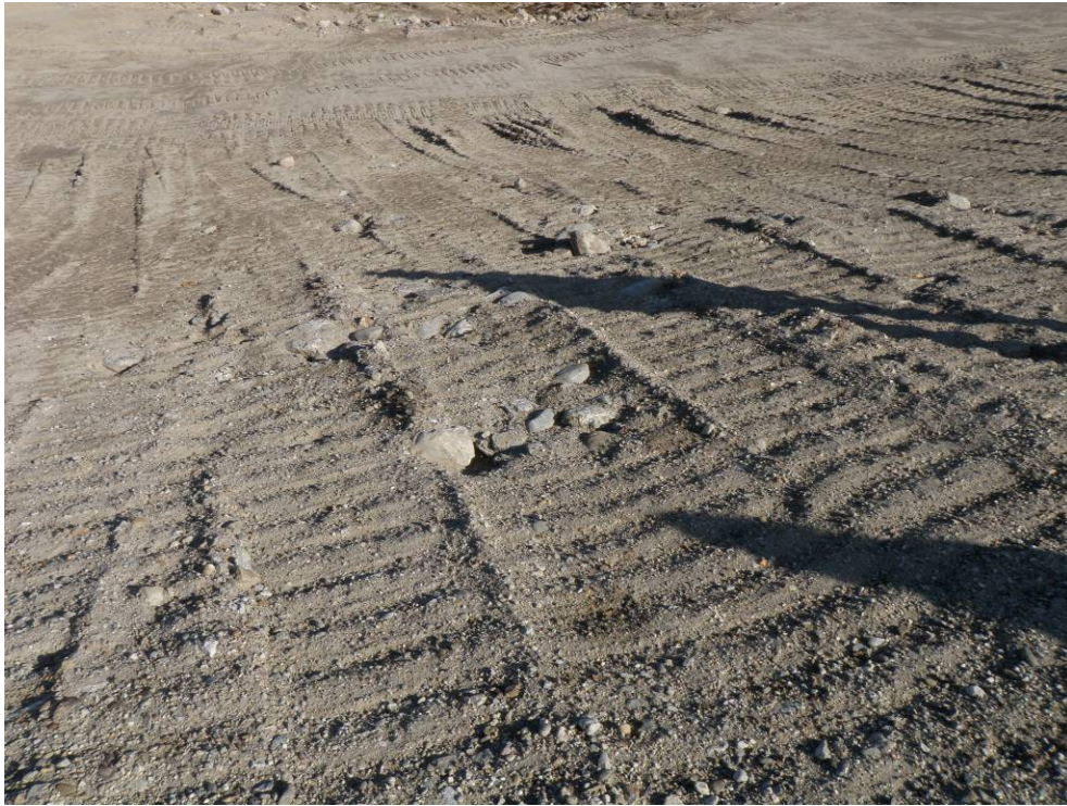
Photo 3. Close-up of eastern side of NHWL showing a few small potholes and exposed cobbles; picture viewpoint number 52 (Figure A-1, Appendix A). Direction photo taken: NE (P8270464).
