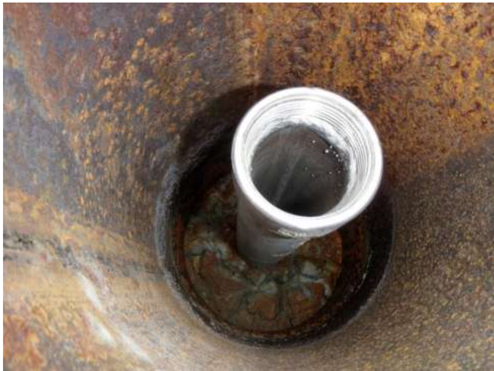
Inside casing of MW-South. Note the bentonite uprising. Viewpoint N/A. Photograph reference 80 (CD-ROM). Direction photo taken: N/A
