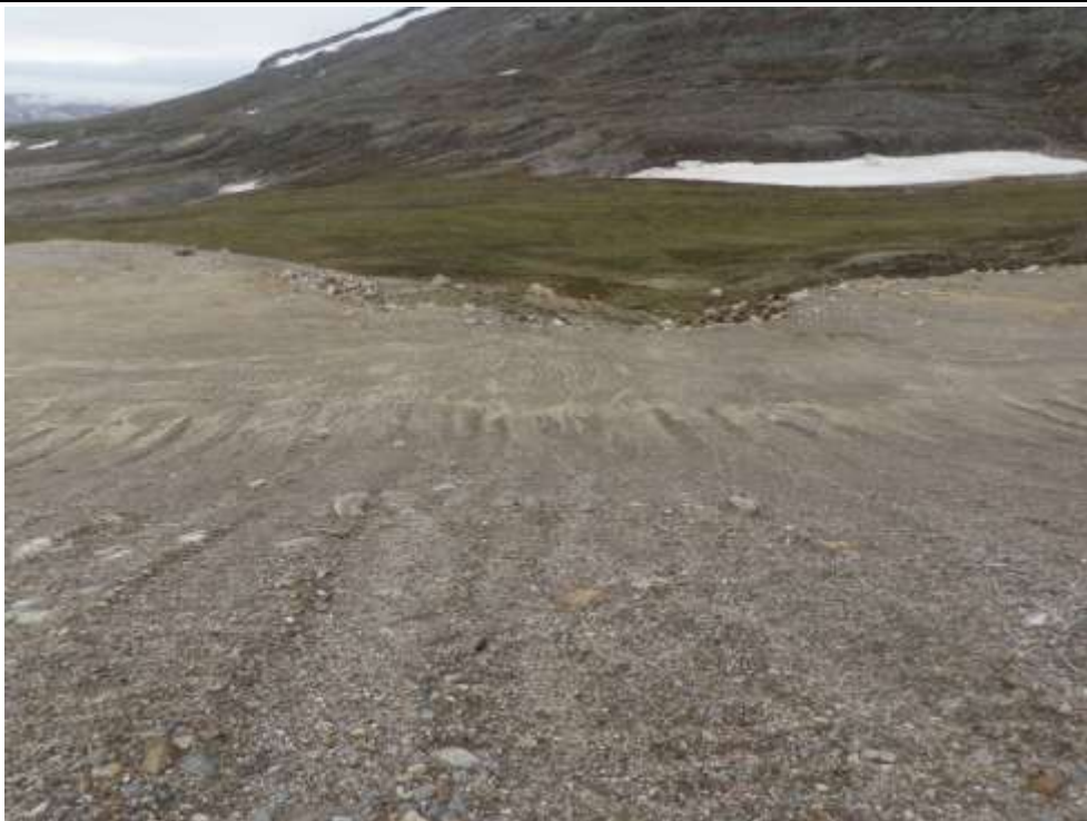
Northeast side of NHWL. Note the erosion channels. Viewpoint 50 (Figure A-1; Appendix A). Photograph reference 50 (CD-ROM). Direction photo taken: NE
