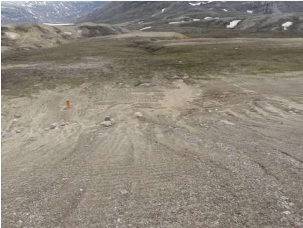
Southwest edge of the landfill. Monitoring well MW-Southeast is at the toe of NHWL. Note the erosion channels. Viewpoint 46 (Figure A-1; Appendix A). Photograph reference 10 (CD-ROM). Direction photo taken: SW
