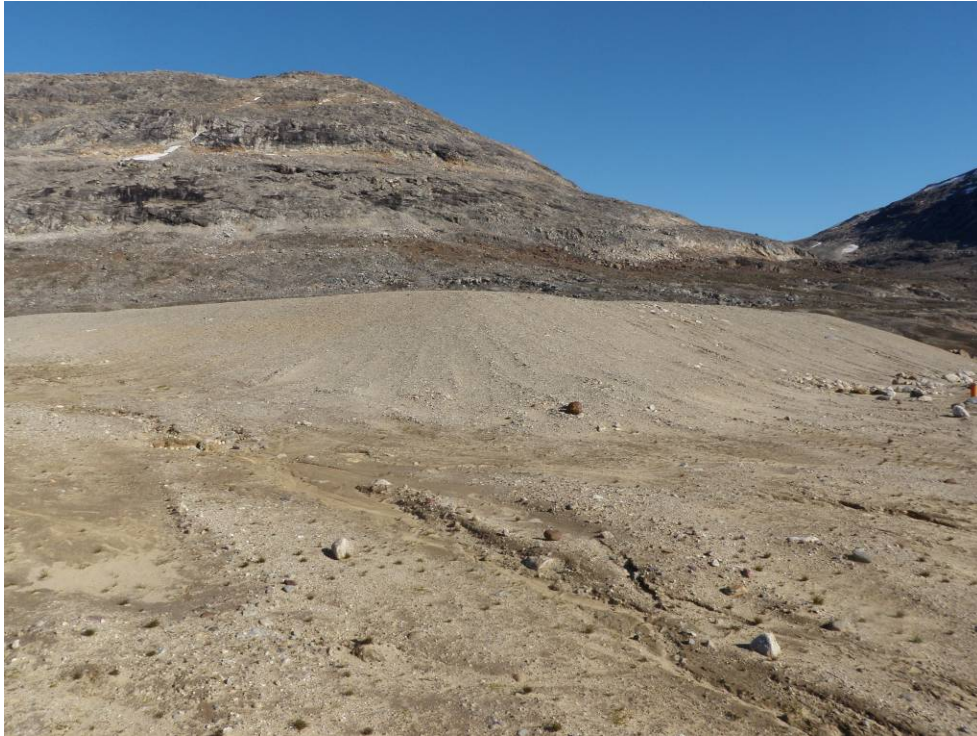
West corner of the NHWL. Note the erosion channel at the toe of the NHWL. Viewpoint 19 (Figure A-1; Appendix A). Photograph reference 19 (CD-ROM). Direction photo taken: SE
