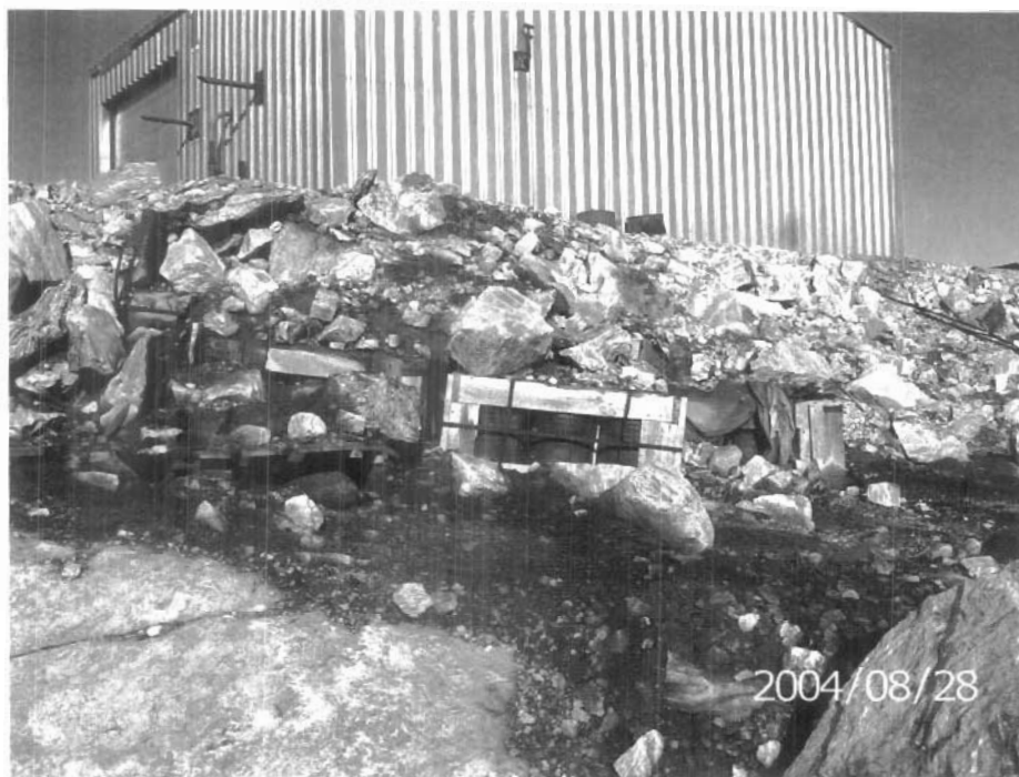
Photo 31 Staining below southwest corner of Garage
