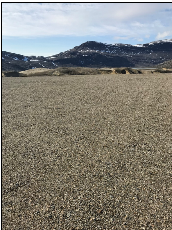
Photograph 11. Top of NHWL, facing west. Cap appears to be very flat with no obvious signs of settlement or depression. No ponded water present.
