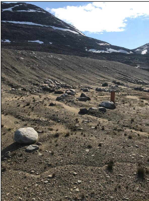
Photograph 4. Runnelling along western edge of NHL, facing southeast. MW-Northwest in view.
