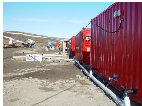
Easily accessible wastewater outlet and piping
