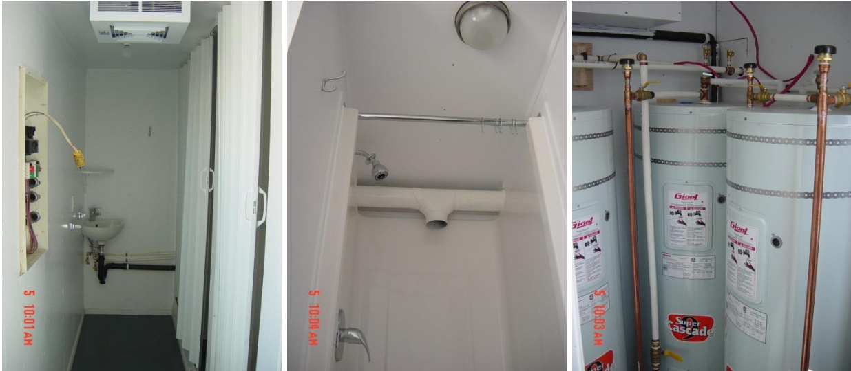
Typical 5 showers / 1 corner wash basin container with: 1 x 2000 watts x 250 cfm ceiling fan heater, dressing room, ventilation and marine light in each shower, 3 x 60 gallons hot water tank, 1 smoke detector and 1 fire extinguisher.
