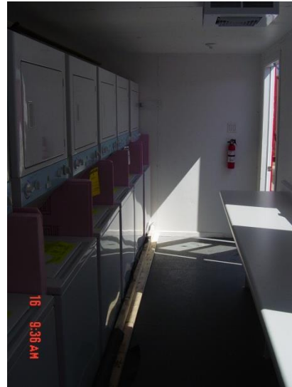
Typical 6 washers/dryers container with: 1 x 2000 watts x 250 cfm ceiling fan heater, 1 x 60 gallons hot water tank, 1 smoke detector and 1 fire extinguisher.
