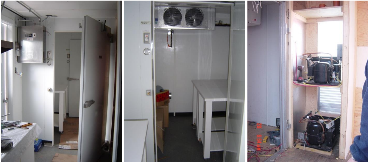
The walk-in fridge (6'x7') and freezer (6'x7') are installed at the back of the kitchen and the compressor units are easily accessible for repair and maintenance
