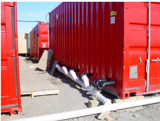
Easily accessible wastewater outlet and piping
