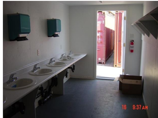
Typical dry room container with: 2 x 2000 watts x 250 cfm ceiling fan heater, 1 x 60 gallons hot water tank, 6 wash basins, 2 paper towel distributor, 1 smoke detector and 1 fire extinguisher.
