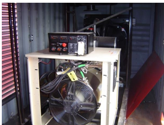
Typical 250 kW generator with associated electrical distribution container
