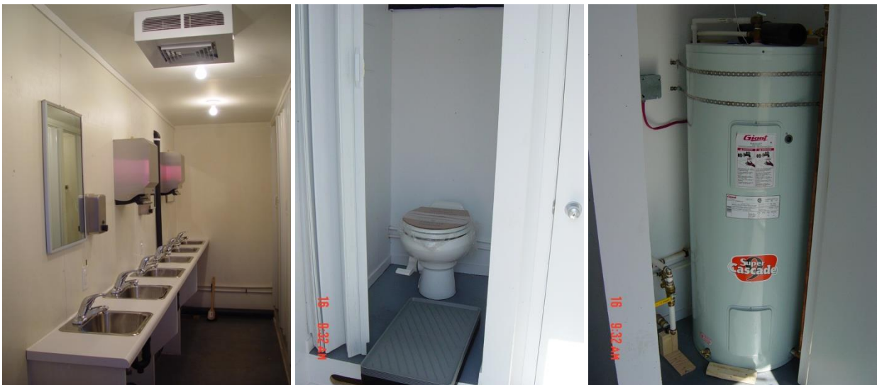
Typical 5 toilets / 2 urinals / 6 wash basins container with: 1 x 2000 watts x 250 cfm ceiling fan heater, 1 x 60 gallons hot water tank, 2 paper towel distributors, ventilation in each toilet and marine light in each toilet, 1 smoke detector and 1 fire extinguisher.
