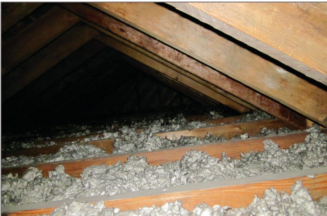
Photo H-38: APEC 18 - Building 5 - Fibre glass insulation (not containing asbestos)
