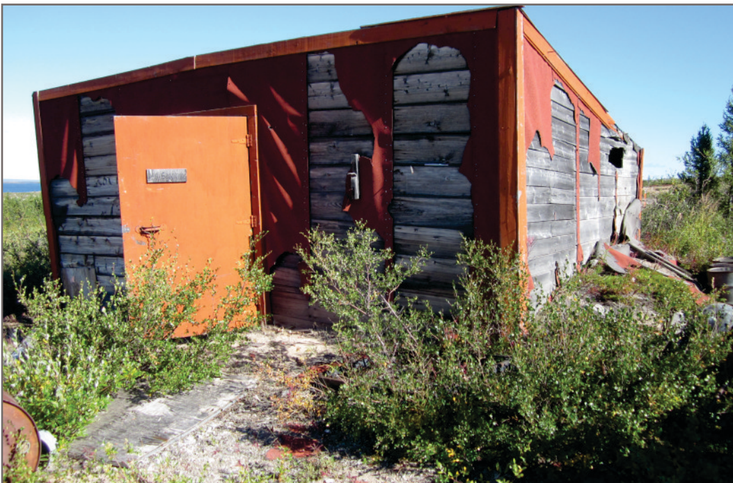
Photo H-40: APEC 20 - Building 7 - Asbestos exterior asphalt shingles and total lead and leachable lead painted wood
