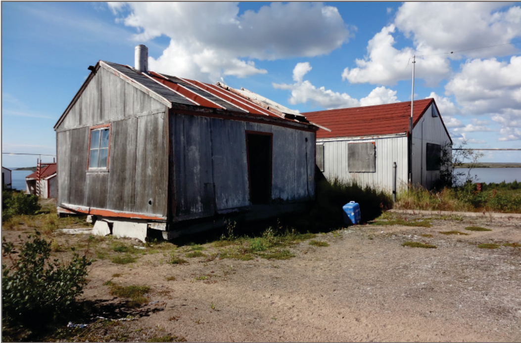
Photo H-31: APEC 17 - Building 4 - Asbestos black felt, attic insulation, window caulking, walls panels and total lead and leachable lead painted wood
