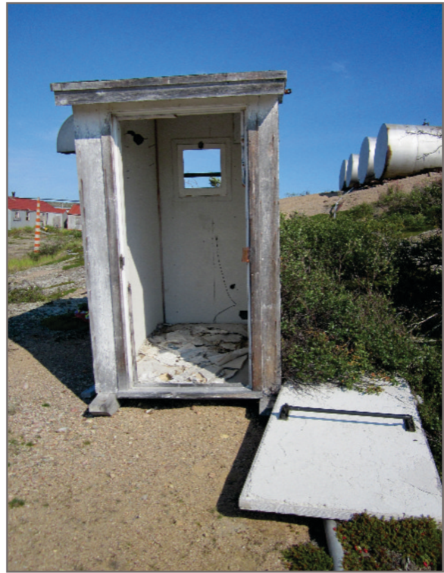
Photo H-5: APEC 7 - Small Cabin - Asbestos black felt and panels, and total and leachable painted wood
