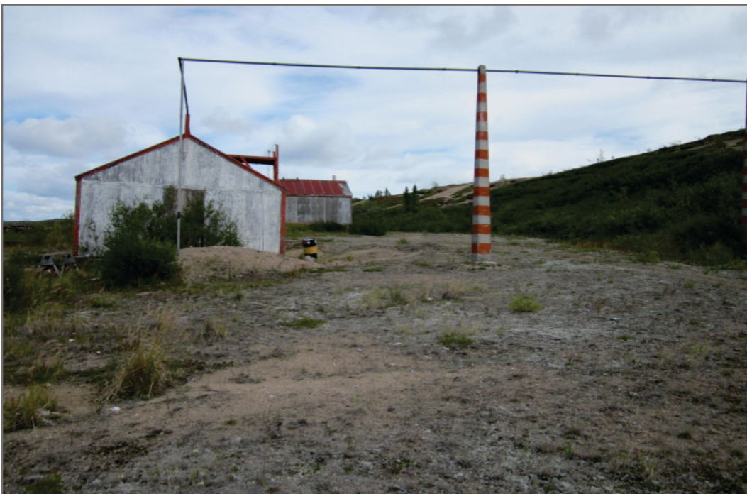
Photo H-10: APEC 13 - Overhead piping from tanks to Buildings - View of overhead piping towards Building 3; total and leachable lead painted concrete and organic content in pipeline
