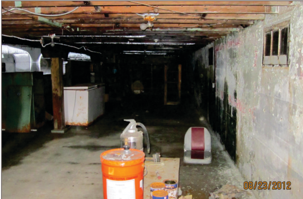
Photo H-13: APEC 14 - Building 1 - Basement total lead and leachable lead painted concrete walls, miscellaneous chemicals, ODS in freezer, mould on wood beams and concrete
