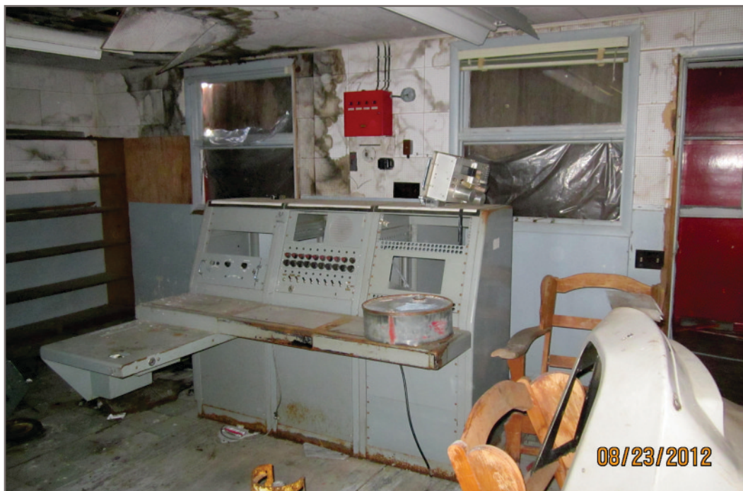
Photo H-21: APEC 14 - Building 1 - Main floor control desk; asbestos walls and ceiling, PCBs, mercury and lead solder in electrical parts
