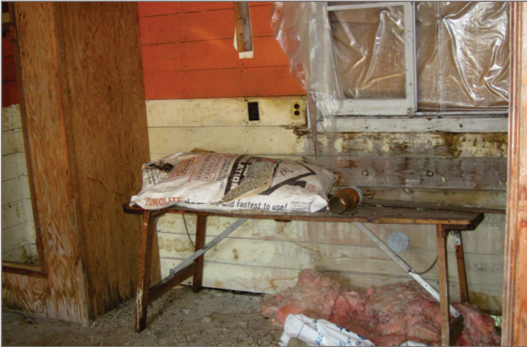
Photo H-33: APEC 17 - Building 4 - Asbestos insulation, and total lead and leachable lead painted wood
