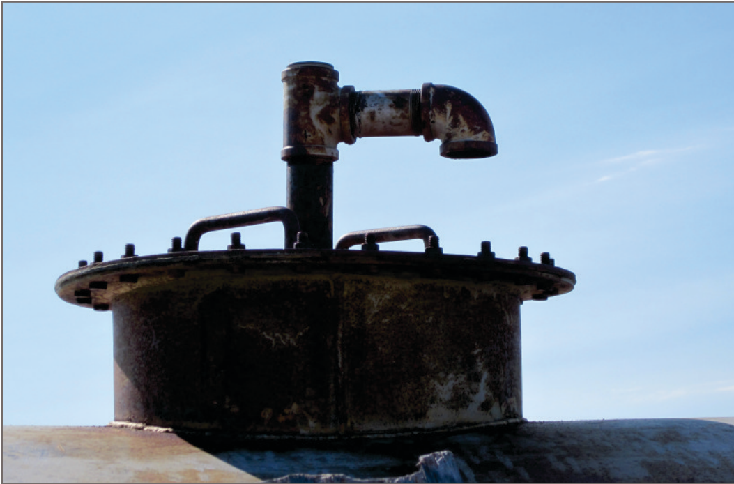
Photo H-9: APEC 9 - Tank 1 - Close-up of asbestos gasket
