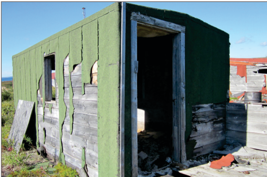
Photo H-42: APEC 21 - Building 8 - Asbestos exterior asphalt shingles and black felt
