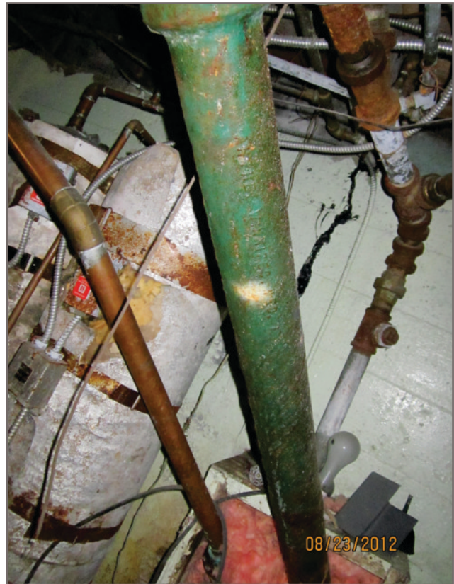
Photo H-17: APEC 14 - Building 1 - Leachable lead seals on cast iron piping and tanks behind
