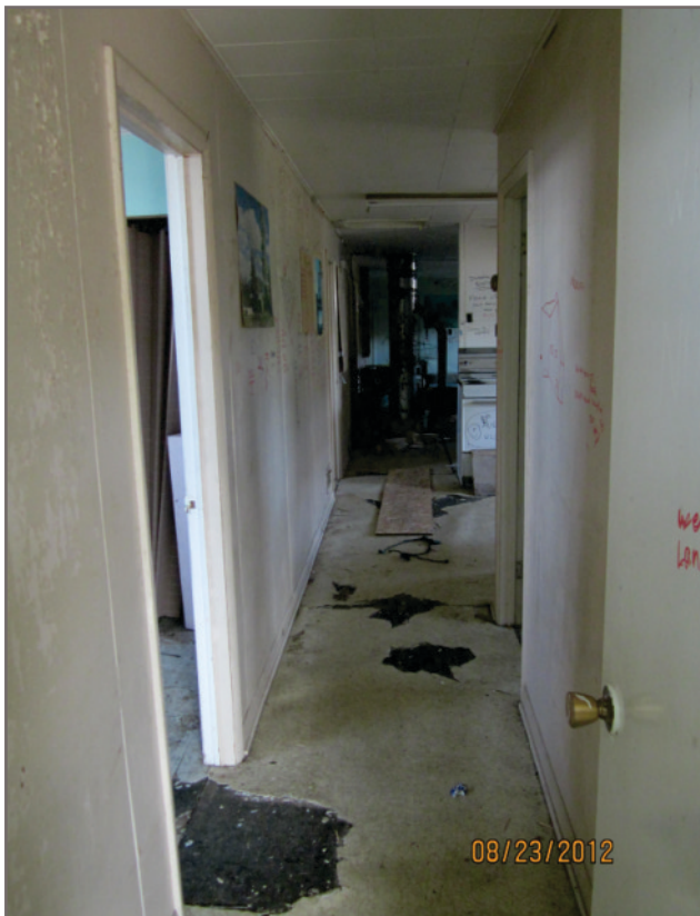
Photo H-18: APEC 14 - Building 1 - Main floor hallway, viewing northeast; asbestos flooring wall panels and ceiling, total lead and leachable lead painted asbestos panels on walls and second layer of ceiling particulate board
