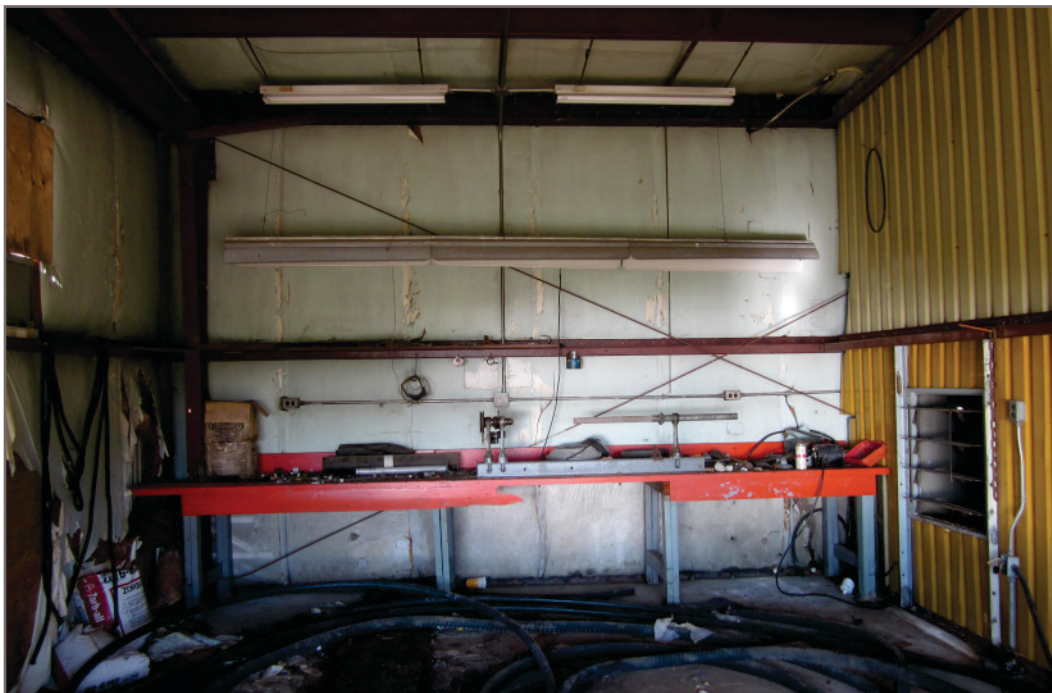
Photo H-25: APEC 15 - Building 2 - Northwest half of building; total lead and leachable lead painted metal walls, ceiling and concrete floor, mercury in lights and PCBs in light ballasts
