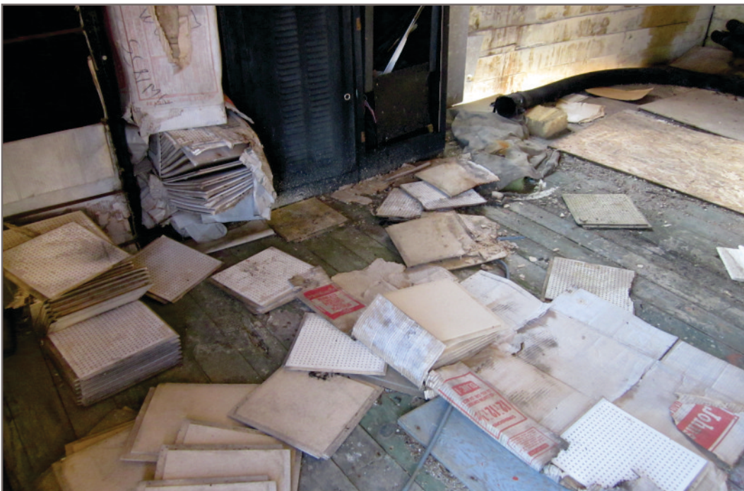
Photo H-32: APEC 17 - Building 4 - Asbestos chimney tile and ceiling tile, and total lead and leachable lead painted wood
