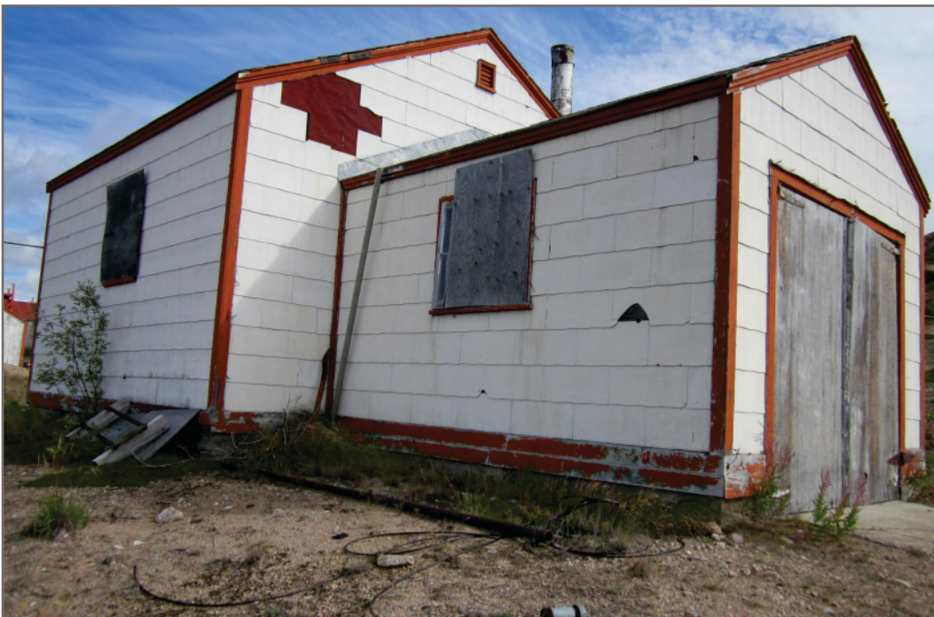
Photo H-34: APEC 18 - Building 5 - Asbestos exterior panels, black felt, attic insulation, window caulking, and total lead and leachable lead painted wood
