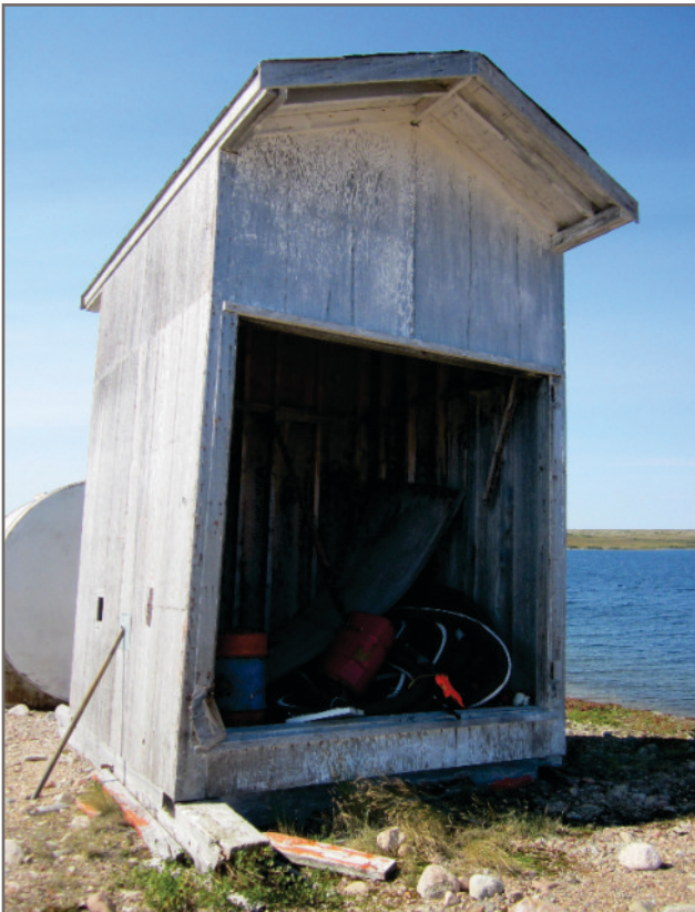
Photo H-4: APEC 6 - Medium Cabin - Asbestos black felt, total lead and leachable lead painted wood exterior and drums and lubricants
