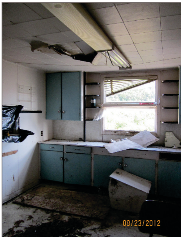
Photo H-19: APEC 14 - Building 1 - Main floor kitchen; asbestos flooring, wall panels and ceiling, total lead and leachable lead painted wood shelves, mercury vapor in lights and PCBs in light ballasts
