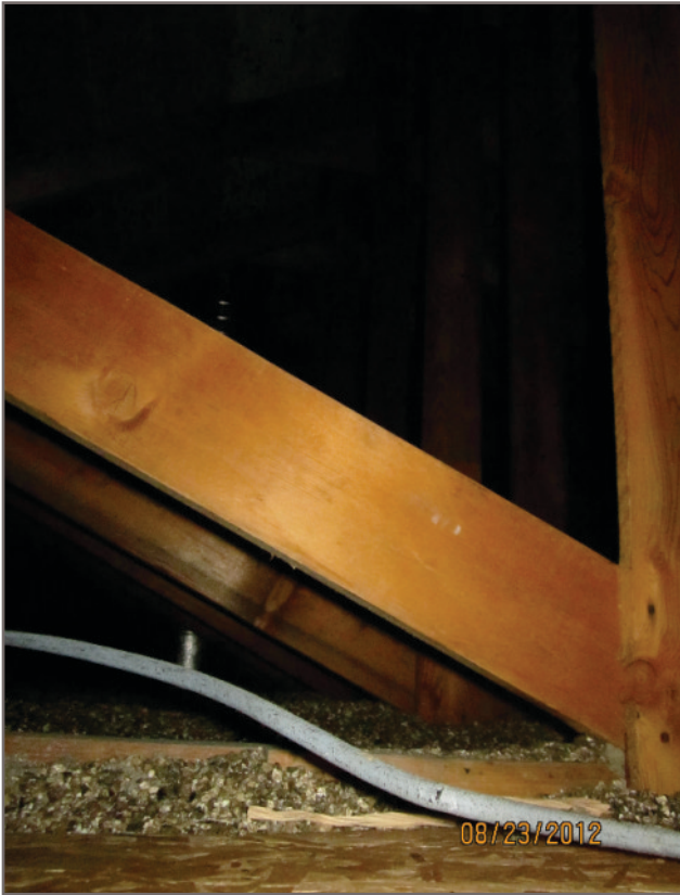
Photo H-23: APEC 14 - Building 1 - Asbestos attic insulation
