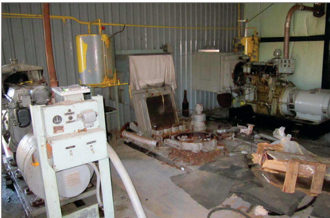
Photo H-26: APEC 15 - Building 2 - Total lead, leachable lead and PCBs painted generators, total lead, leachable lead and PCBs painted plastic over fibreglass insulation, ceiling and concrete floor miscellaneous fluids in generators and lead acid batteries
