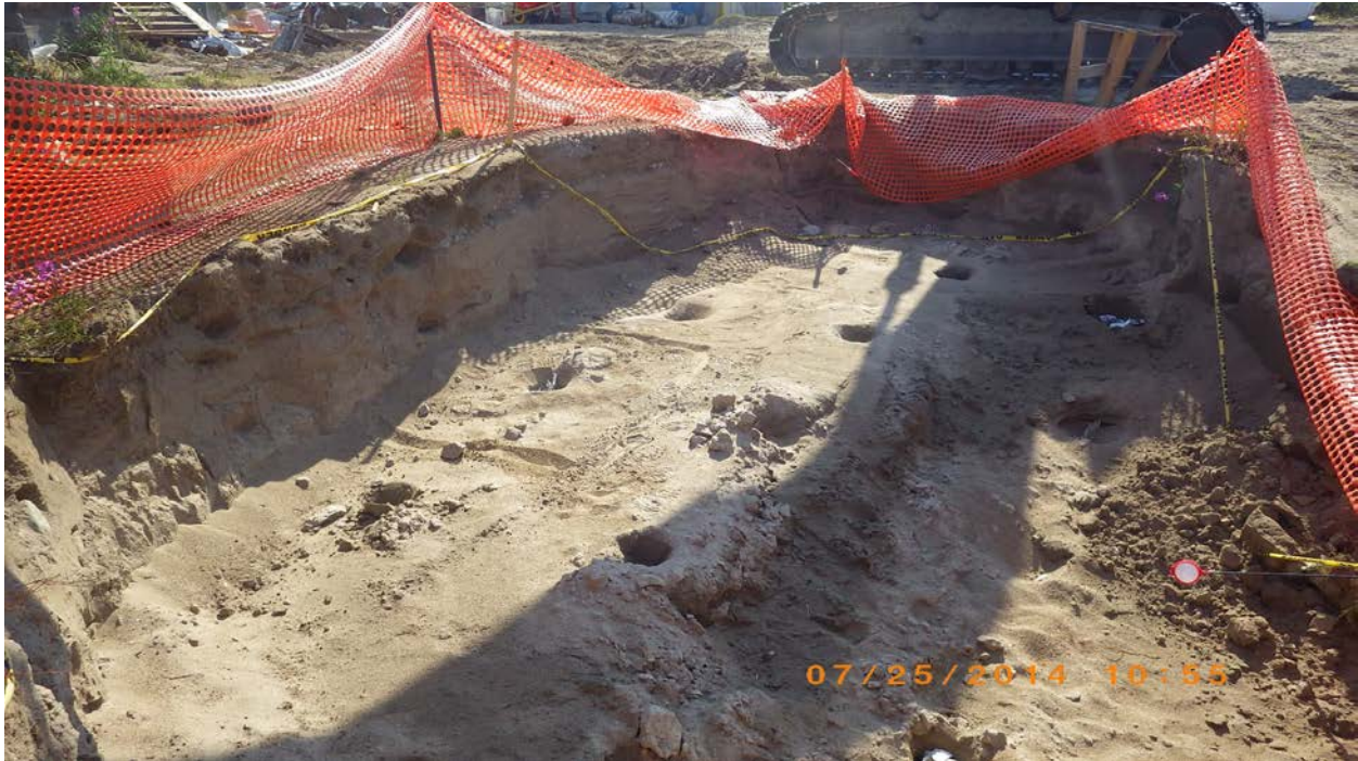
Photo 25: Looking south over APEC 13.1 excavated to survey limits. Note square on left hand side indicating sample exceedance that was further excavated (July 25, 20114).
